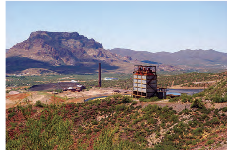
Historical Magma Mine workings and the smelter complex
