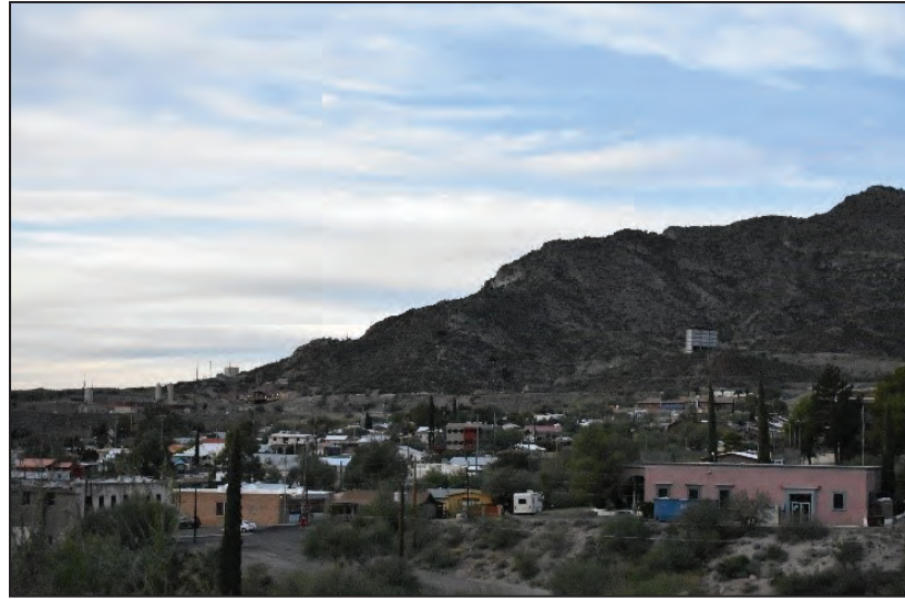
View overlooking the town of Superior and the West Plant Site
