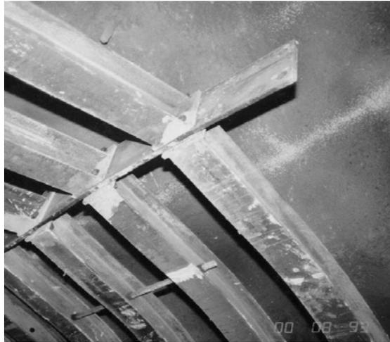
**Figure 5a : Connecting plate**
