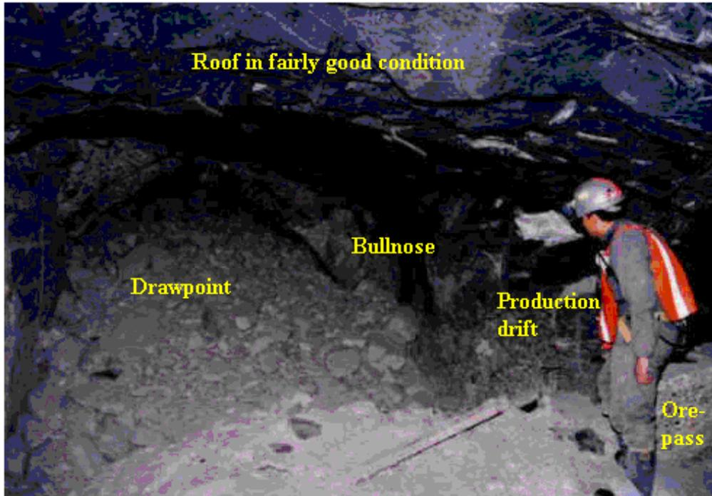
**Collapsed area with sidewall failure**
