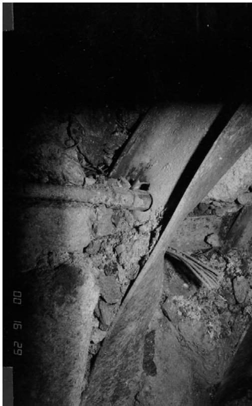
**Figure 9 : Failed connecting rod between the rigid 'H' profile arches.
