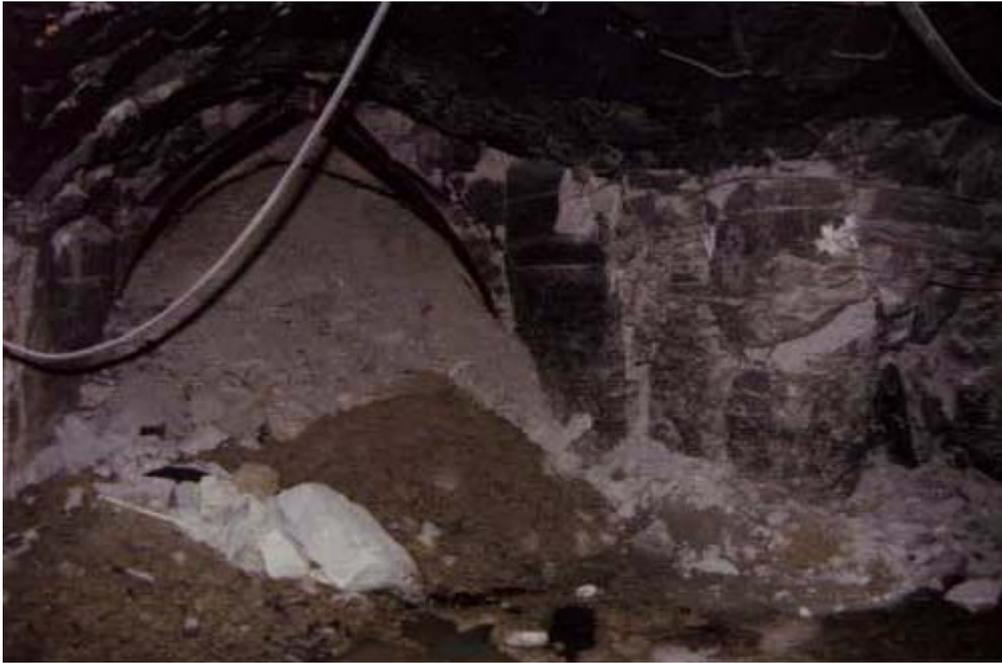
At Shabanie Mine modelling showed that there should be high stress effects in the perimeter of a 110m by 120m opening, but nothing unusual was noted, as stress relief occurred with very small movements on joints in the surrounding rock mass.
