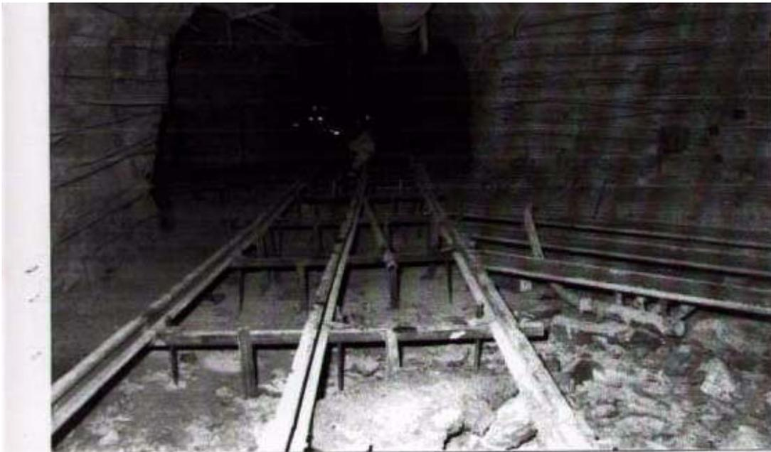
**P.5.3. Footwalls were supported with a rail construction bolted into the footwall encased in at least 500mm of concrete to provide good roadways for LHD trammin**
