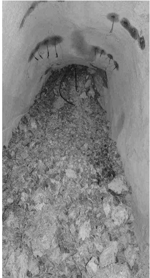
**Figure 4** Pneumatic loading of ANFO explosives on the left and charged and primed holes ready for blasting on the right
