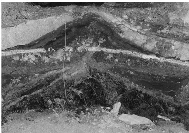
**Cross section through a floor that has heaved**
