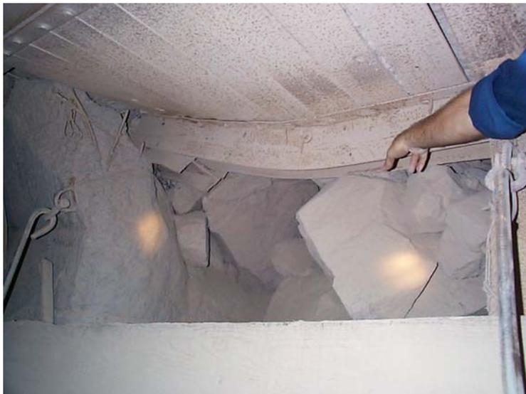
**Concrete brow has failed and the steel repair beam is taking ‘weight’**
