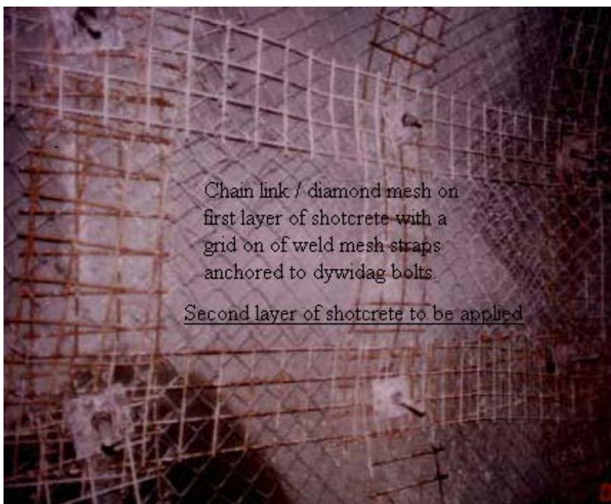
**Heavy duty weld mesh straps on chain link mesh, anchored by dwyidag bolts**
