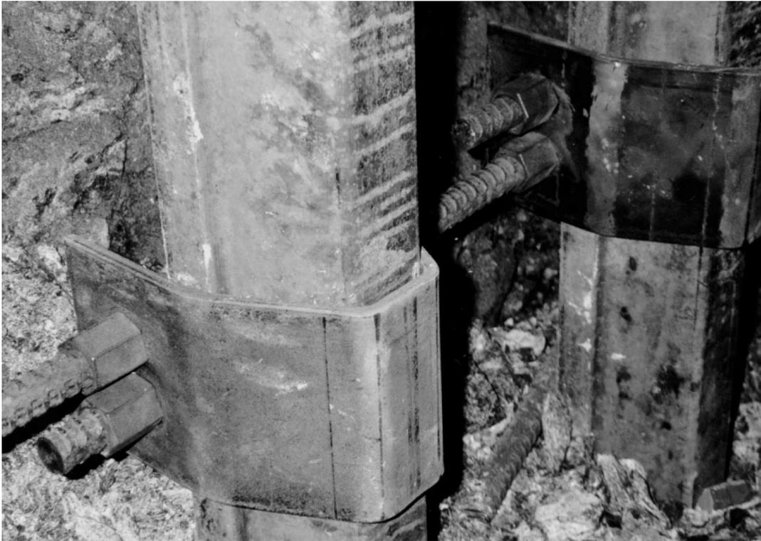
**Figure 8 : New system offered flexibility and strength to the yielding arches**
