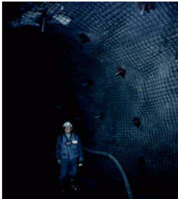
On those mines using diamond / chain link mesh there is no difficulty in shotcreting the mesh when done by competent personnel. This photograph shows that shotcrete can be placed in tight areas if the support installation procedure demands that this should be done. There are no excuses for poor workmanship.
