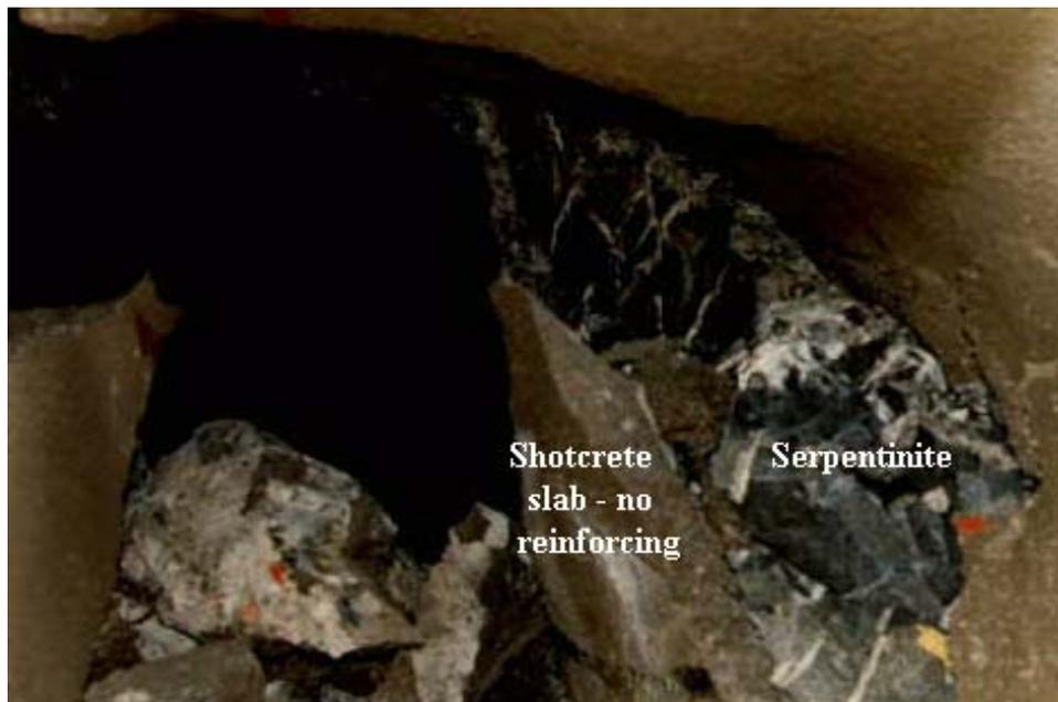
**Shotcrete without reinforcement fails at low deformation**
