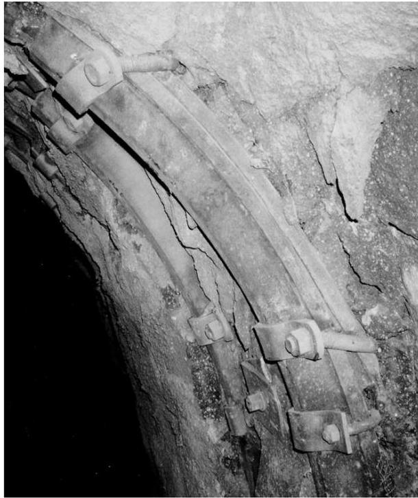
**Figure 10a : Failed 'U' clamp -yielding arch**
