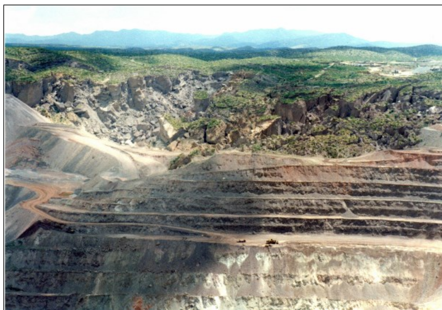
Figure 6 17 Open pit at San Manuel, looking south toward Santa Catalina Mountains on skyline. Broken ground in the far wall resulted from the collapse of surface exposures above the underground block caving operation.
