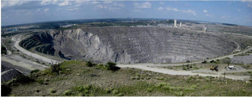
Figure 15. Palabora mine pit. Caved area from UG block caving operations on the left.
