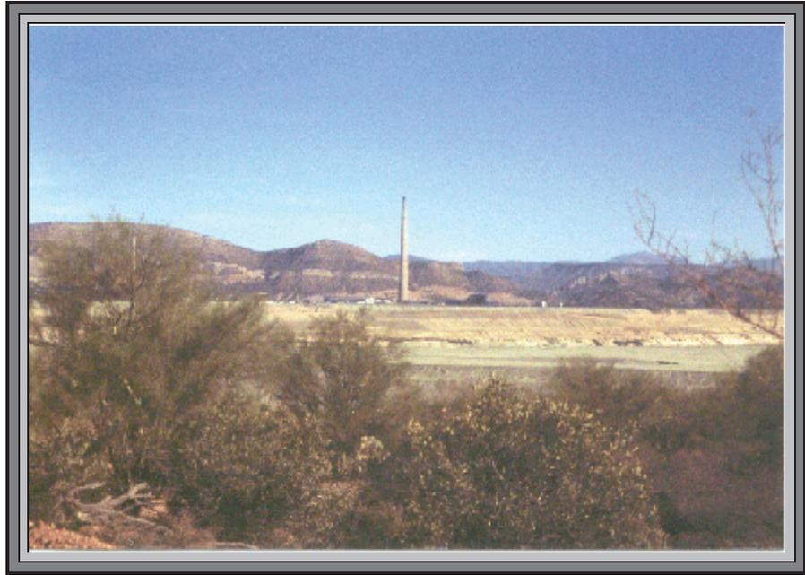
Figure 8. The San Manuel copper mining complex, including the smelter smokestack and tailings piles are shown in this photo. Groundwater from the underground mining operations had been pumped at a rate of 4,000 gpm and applied to the tailings piles for dust control. This practice ended in January 2002 when a four inch cover of rock material capped the more than 3,000 acres of tailings dumps<sup>23</sup>.
