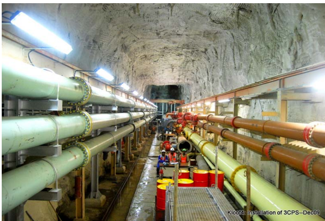
Figure 3. Typical hydro-displacement station
