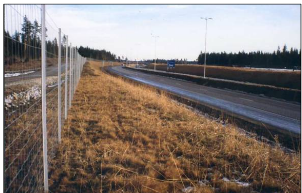
Figure 9: Potential road mitigations (from top to bottom) include: highway overpasses, bridges, culverts, and drainage pipes. Fencing (lower right) should be used to guide animals into crossing structures.
