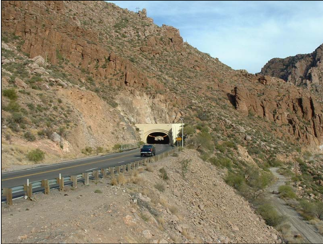
Figure 7: East (azimuth 68) from waypoint 109, US-60 runs through a tunnel for about 375 meters. The rocky “wildlife bridge” above the tunnel is an ideal crossing structure for bighorn sheep.
