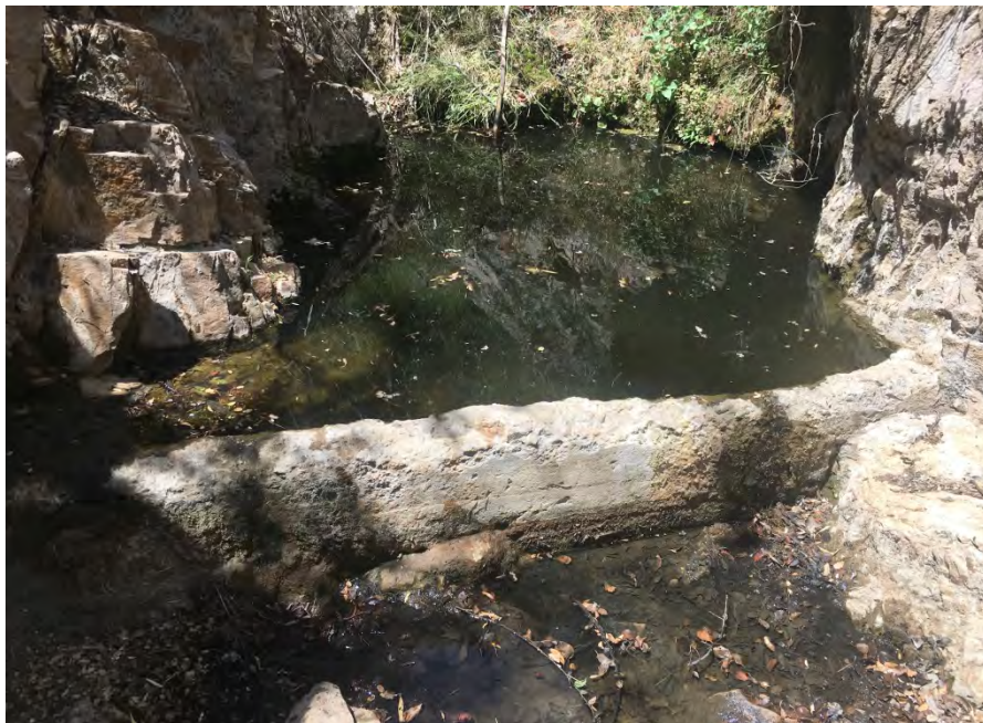
PHOTO 4b. Chimney Spring; concrete headwall in quartzite; June 2018.
