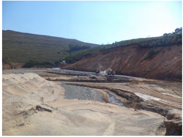
MISC-H: Photo from morning on day of failure from eyewitness report, November 5, 2015, showing toe of El. 860 m blanket drain.
