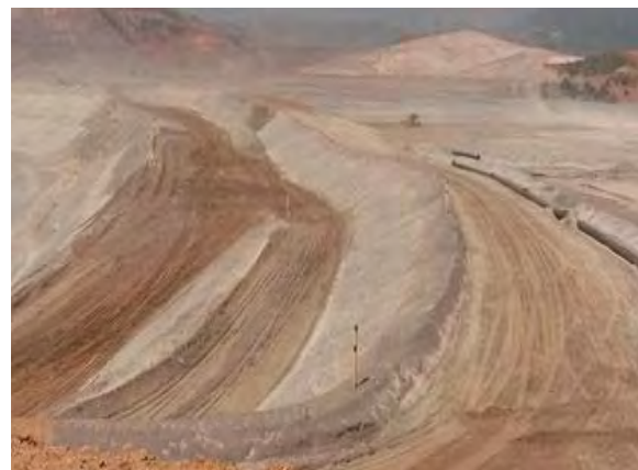
20-A: Photo from weekly report, week of October 4, 2015: "3 m widening downstream, between piles 27 to 41, at the left-side abutment, for crest heightening to 900 m."
