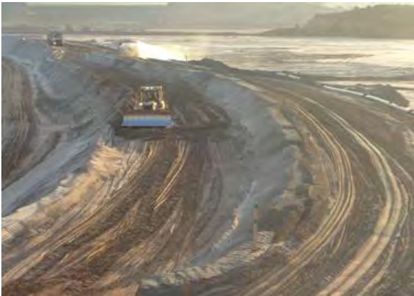
20-E: Photo from weekly report, week of October 11, 2015: "Heightening of the crest, downstream, to elevation 899.00 m, left-side abutment."
