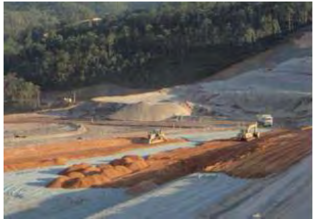
10-A: Photo from weekly report, week of June 28, 2015: "Construction of drain carpet on the left-side abutment of Dike 1."
