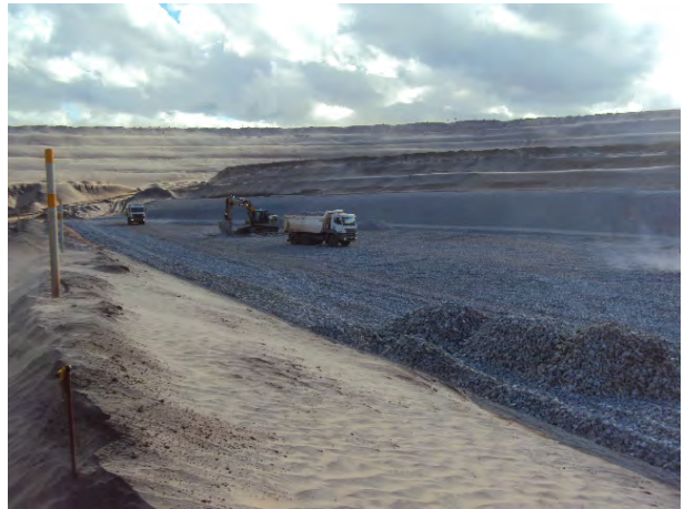
10-I: Photo from Technical Monitoring Photographic Report (2015-06-29 to 2015-07-03) [19] showing drain rock placement on left setback.
