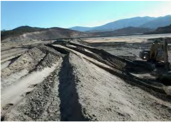
16-E: Photo from weekly report, week of September 13, 2015: "Extension of the pipeline, positioning of the cannon and discharge of the Plant 3 sand tailings into Bay "C", Dike 1, to ensure the shore width (minimum of 200 m)."
