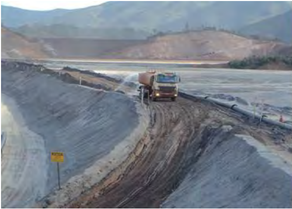
3-A: Photos from weekly report, week of May 31, 2015: "Construction begin of the 25.00 m plateau upstream at, to the 890 m elevation. At Dike 1."
