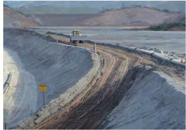
3-A: Photos from weekly report, week of May 31, 2015: "Construction begin of the 25.00 m plateau upstream at, to the 890 m elevation. At Dike 1."
