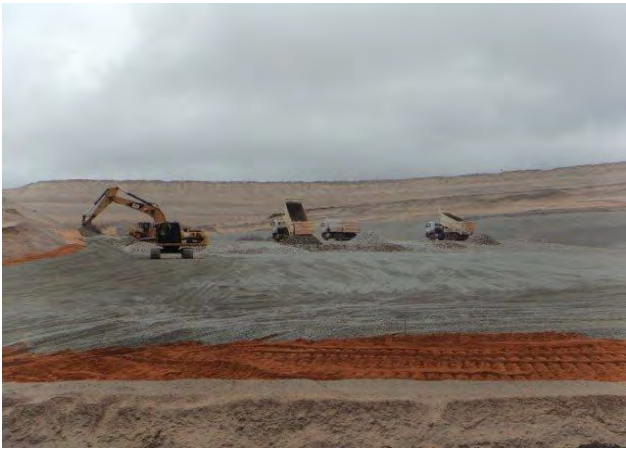
4-A: Photo from weekly report, week of June 14, 2015: "Construction of a drainage blanket on the left-side abutment of Dike 1."
