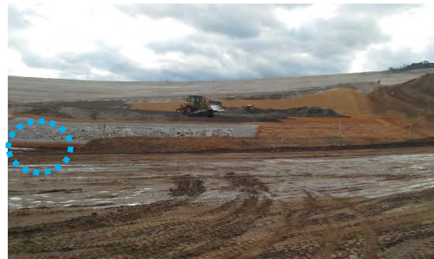
14-B Samarco construction photo from August 10, 2015 showing drain construction on the left setback.
