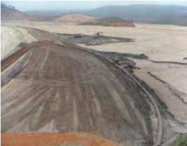
8-A: Photo from weekly report, week of June 28, 2015: "Heightening of the platform upstream from bay C, near PL1 cannon."
