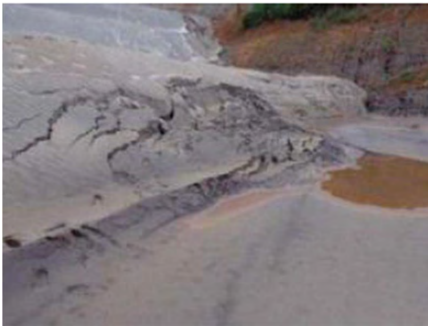
Figure 2-11 November, 2013 seepage, cracking, and slumping at left abutment El. 860 m
