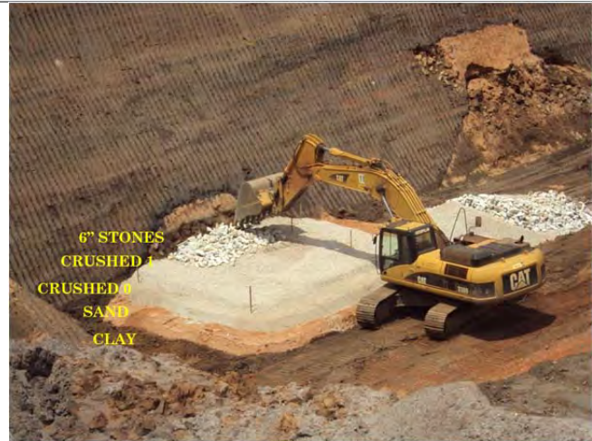
October, 2010 construction photo showing plugging of the Auxiliary Foundation Drain to the left with the excavated Principal Foundation Drain to the right.
