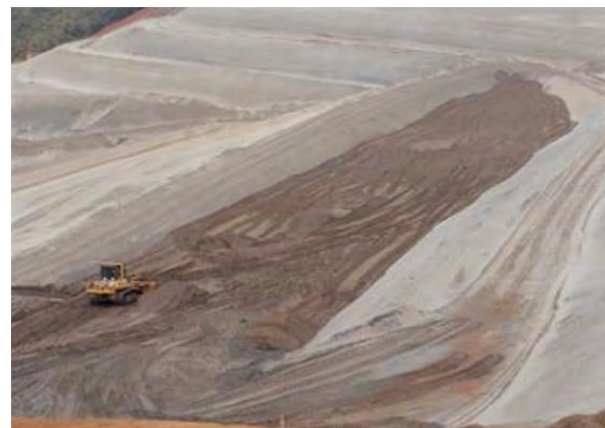
19-B: Photo from weekly report, week of October 25, 2015: "Preparation of the axis return area for hydraulic discharge."
