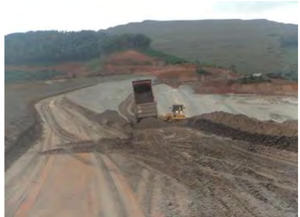
16-B: Photo from weekly report, week of September 6, 2015: "Heightening of the 890.00 m bank."
