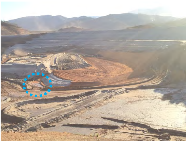
14-G: Samarco construction photo from August, 2015 (exact date unknown) showing left setback. Dashed blue line around ponded water.
