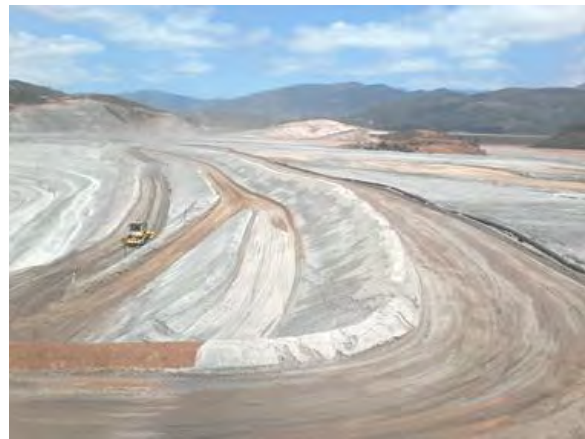
16-G: Photo from weekly report, week of September 13, 2015: "890/895 m elevation leveling to allow continuity of the heightening of the return to the original axis of Dike 1, Left-side abutment"
