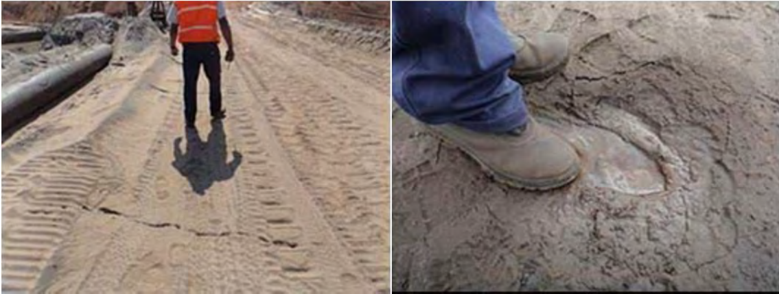
Figure 2-15 Cracks on dam crest and saturation at toe of slope, August 27, 2014
