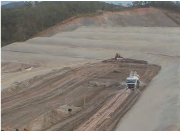
9-D: Photo from weekly report, week of July 5, 2015: "Tailings discharge to recover the original axis of Dike 1."
