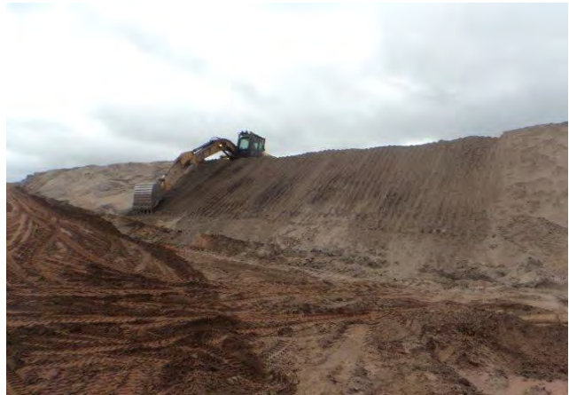
6-C: Photo from weekly report, week of June 14, 2015: "Surface leveling downstream of the 895.0 m bank, on Dike 1."
