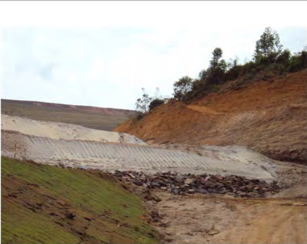
Figure 5.4 ~ Performance of an inverted drain ~ Dike 1 heightening, left abutment.
