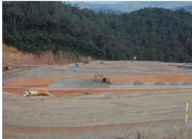
MISC-C: Photo from weekly report, week of May 24, 2015: "Continued construction of blanket drain at the left-side abutment of Dike 1."
