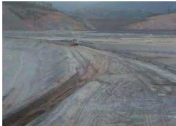
8-D: Photo from weekly report, week of July 19, 2015: "Leveling of the entire extent of the Dike 1 crest."
