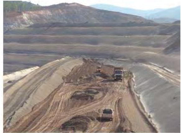
19-A: Photo from weekly report, week of October 18, 2015: "875.00 m bank earthfill for axis return and crest stability."
