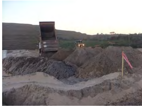
13-A, B: Photos from weekly report, week of August 2, 2015: "Heightening of the crest of Dike 1, phases 1 and 3, to the 895.50 m elevation, piles 6 to 20."
