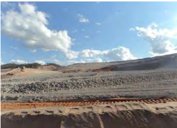
10-F: Photo from weekly report, week of July 5, 2015: "Construction of drain blanket on the left-side abutment of Dike 1."
