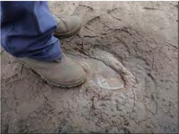
September 2014 inspection photo showing saturation of material at the toe of the El 865 m bench.
