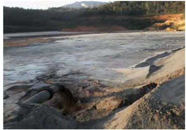
16-E: Photo from weekly report, week of September 13, 2015: "Extension of the pipeline, positioning of the cannon and discharge of the Plant 3 sand tailings into Bay "C", Dike 1, to ensure the shore width (minimum of 200 m)."
