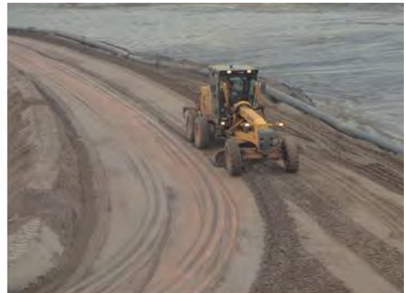
16-C, D: Photo from weekly report, week of September 6, 2015: "Tanker truck and power grader to water and level the 898.00 m crest, near the left-side abutment channel."
