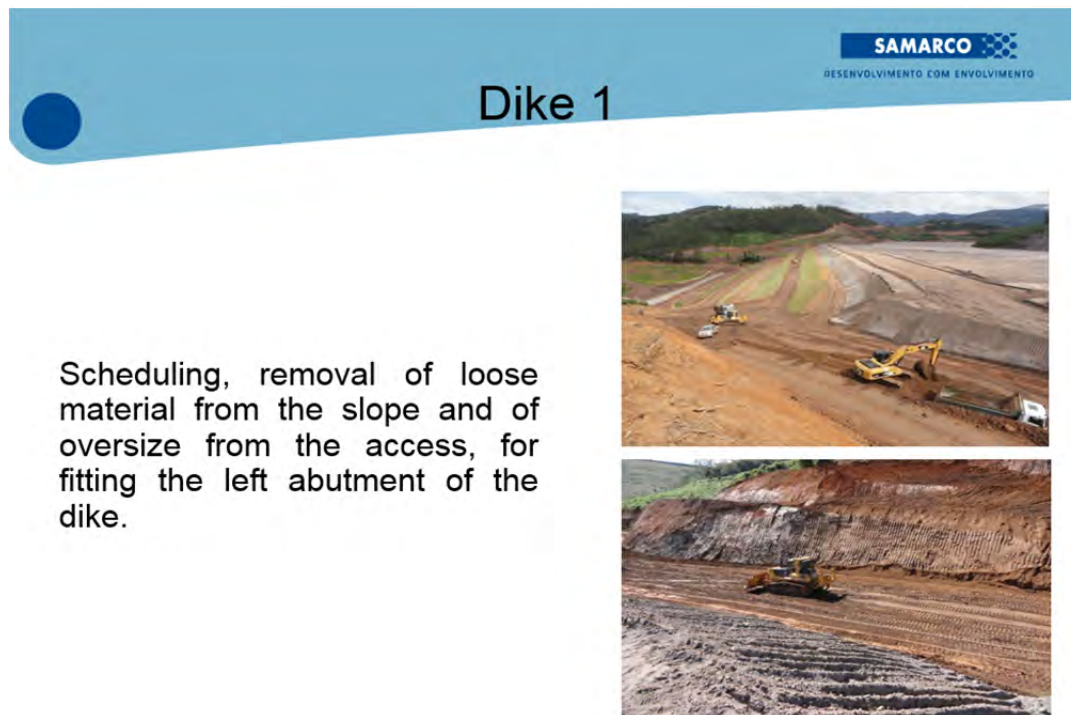
Figure B5-20 Photos of ground preparation prior to upstream raise from weekly report dated May 21-27, 2012
