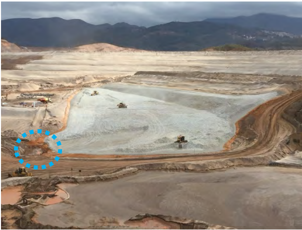
10-H: Photo from Technical Monitoring Photographic Report (2015-06-29 to 2015-07-03) [19] showing left setback. Dashed blue line around ponded water.
