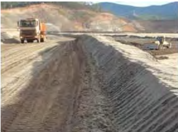
6-F: Photo from weekly report, week of June 21, 2015: "Elevation of phase 4 to allow the elevation of the 900 m bank, Dike 1."
