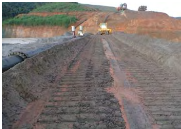
3-C: Photo from weekly report, week of June 7, 2015: "Spreading and compaction of the tailings on the left-side abutment."
