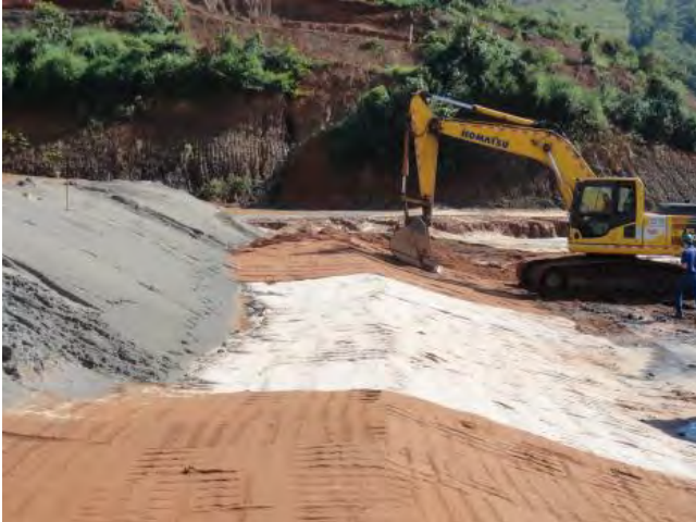
Photo from December 23-29, 2013 weekly report showing placement of sand over area of upwelling.
