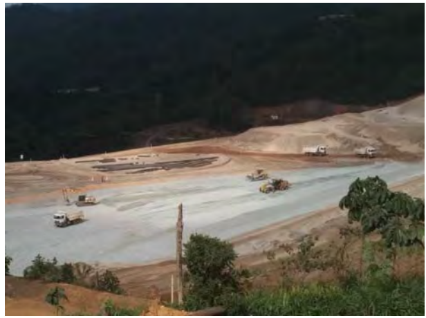
10-C: VOGBR photo from July 2, 2015 [18] showing drain rock placement on left setback.
