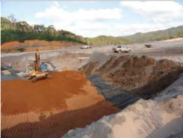
Construction photo from June 17-23, 2013 weekly report showing the geotextile and sand placement, with the beginnings of the rockfill trench to the left.
