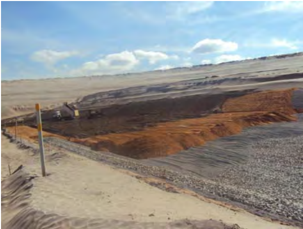
10-J: Photo from Technical Monitoring Photographic Report (2015-07-13 to 2015-07-17) [20] showing sand placement.
