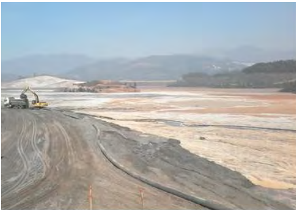
20-C, D: Photo from weekly report, week of October 11, 2015: "Heightening of the berm downstream from the left-side abutment, to ensure a safe height (5.00 m) between banks 895/900 m, allowing the heightening to proceed."
