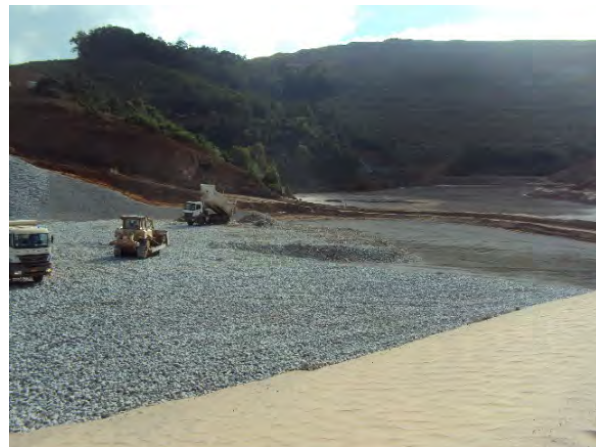
10-G: Photo from Technical Monitoring Photographic Report (2015-06-29 to 2015-07-03) [19] showing drain rock placement on the left setback.
