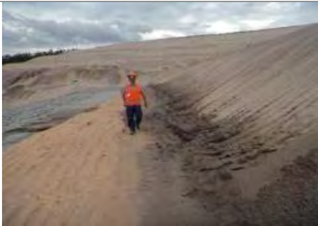
Photo from monthly geotechnical report showing saturation at the toe of the slope above the El. 860 m blanket drain.
