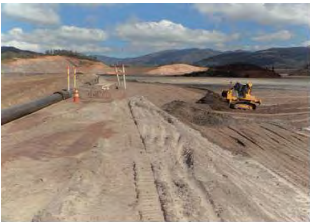
3-B: Photo from weekly report, week of May 31, 2015: "Heightening along the entire crest of Dike 1, finalizing the 895.00 m bank."
