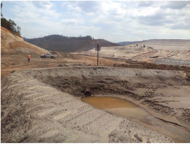
MISC-G: Photo from morning on day of failure from eyewitness report, November 5, 2015, showing toe of El. 860 m blanket drain.
