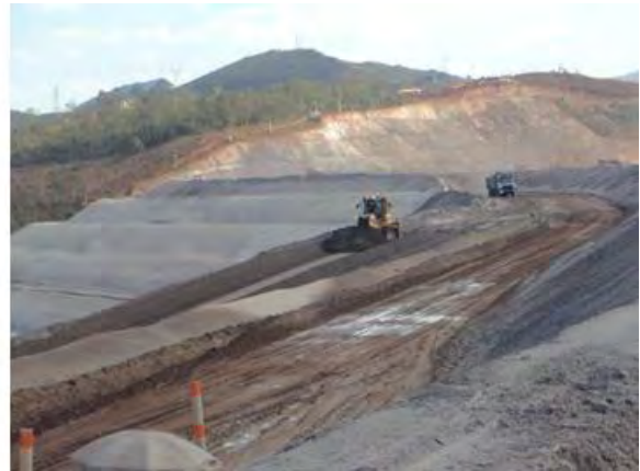
16-H, I: Photo from weekly report, week of September 20, 2015: "Heightening of the axis return in the 890.00 m - 895.00 m bank, left-side abutment of Dike 1."
