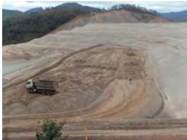
6-E: Photo from weekly report, week of June 21, 2015: "Elevation of the crest at the left-side abutment connection."
