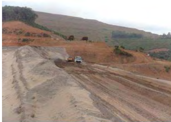
20-F: Photo from weekly report, week of October 24, 2015: "Construction of a reinforcement berm downstream from the 895/900 m bank, on the left-side abutment."
