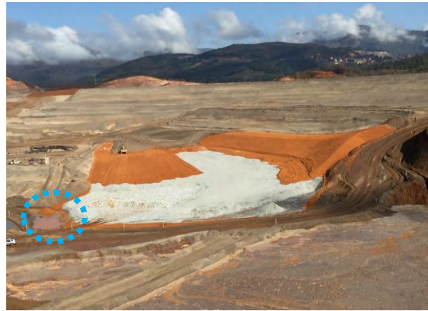
10-E: Photo from weekly report, week of July 5, 2015: "Construction of drain blanket on the left-side abutment of Dike 1." Dashed blue line around ponded water.
