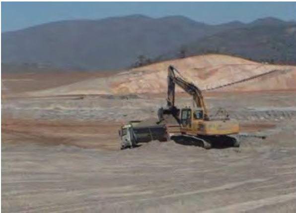
16-H, I: Photo from weekly report, week of September 20, 2015: "Heightening of the axis return in the 890.00 m - 895.00 m bank, left-side abutment of Dike 1."
