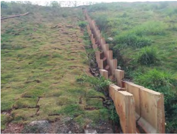
MISC-D: VOGBR photo from July 2, 2015 [18] : "Left Abutment - Saturation in the Slope - El. 826 m."
