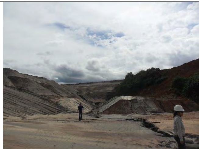
March 27, 2014 site visit photo from VOGBR showing the open channel looking upslope towards the dam crest. The erosion on the setback plateau can be seen to the right of the photo.
