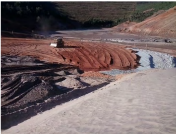
14-C: Samarco construction photo from August 11, 2015 showing drain construction on the left setback.
