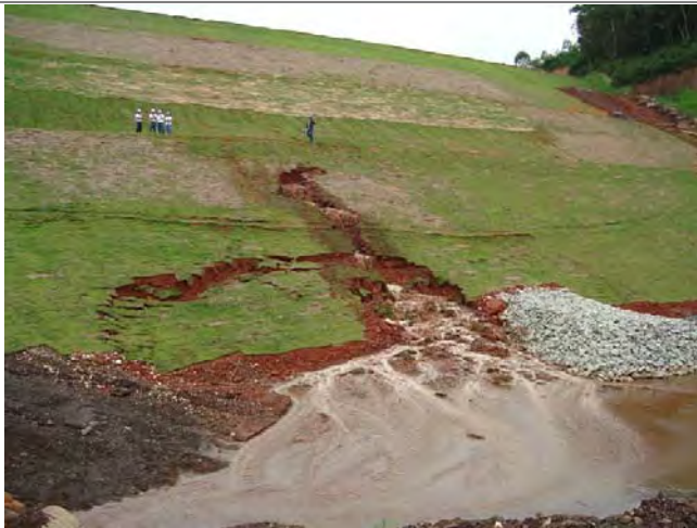
April 13, 2009 site inspection photo [23] showing piping on the downstream face of Dike 1. The Principal Foundation Drain can be seen to the right of the spring.
