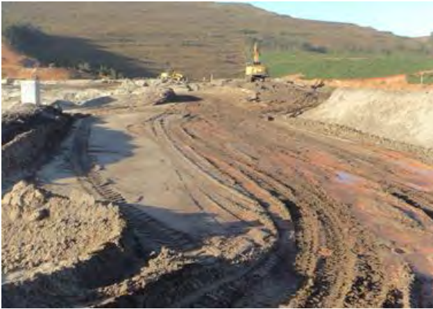
13-A, B: Photos from weekly report, week of August 2, 2015: "Heightening of the crest of Dike 1, phases 1 and 3, to the 895.50 m elevation, piles 6 to 20."
