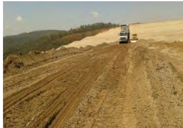
16-K: Photo from weekly report, week of September 27, 2015: "Construction of a dike for tailings to be discharged hydraulically at the original axis, L.S.A., Dike 1."
