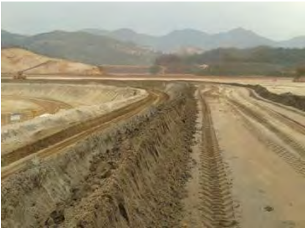
16-L: Photo from weekly report, week of September 27, 2015: "Heightening of the L.S.A. drain protection dike, between piles 1A and 7A."
