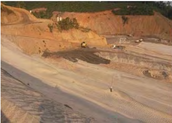
19-A: Photo from weekly report, week of October 18, 2015: "875.00 m bank earthfill for axis return and crest stability."
