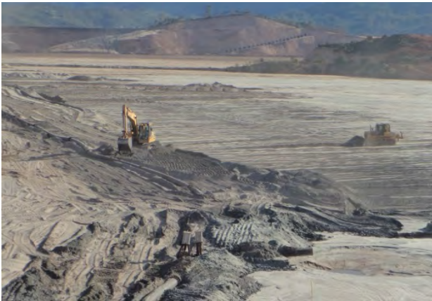
13-C: Photo from weekly report, week of August 9, 2015: "Heightening of the upstream platform, between as piling 20 to 40, to the 896.00 m elevation."
