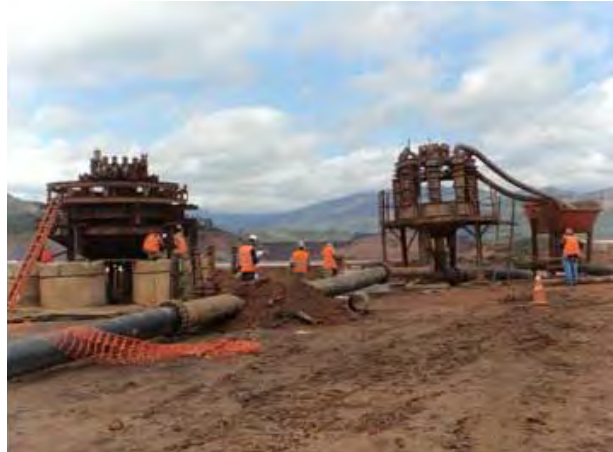
MISC-A: Photo from weekly report, week of May 3, 2015: "Continued hydrocyclone assembly."
