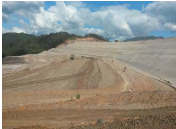
6-A: Photo from weekly report, week of June 7, 2015: "Landfill over the left-side abutment drain, to the 877.0 m elevation."
