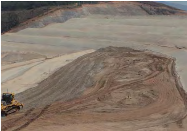
16-J: Photo from weekly report, week of September 20, 2015: "Construction of a dike to form a bay, in the 875.00 m elevation. This activity is to allow the return to the original axis, downstream from the left-side abutment, for controlled hydraulic discharge with minimum outflow."
