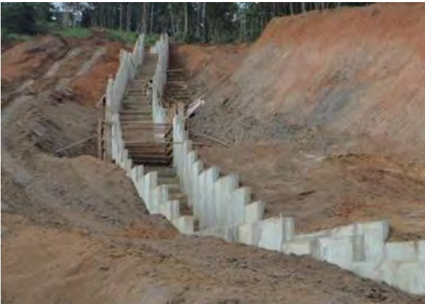
MISC-B: Photo from weekly report, week of May 17, 2015: "Construction of drainage chutes at the left-side abutment of Dike 1."
