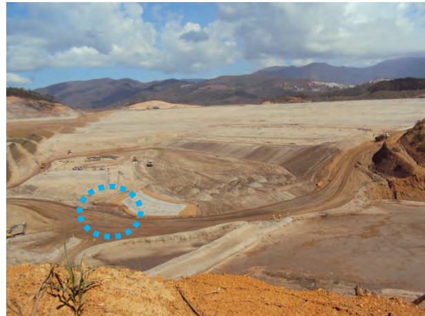
17-A: Photos from VOGBR report dated August 21, 2015 to August 28, 2015 [22] . Dashed blue line around ponded water. Stockpiles could account for increased elevations seen in isopach for August 24, 2015 to October 1, 2015 surveys.
