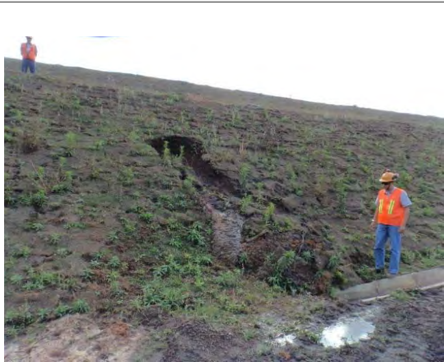
July, 2014 inspection photo showing seepage outbreak on the downstream face of Dike 1.
