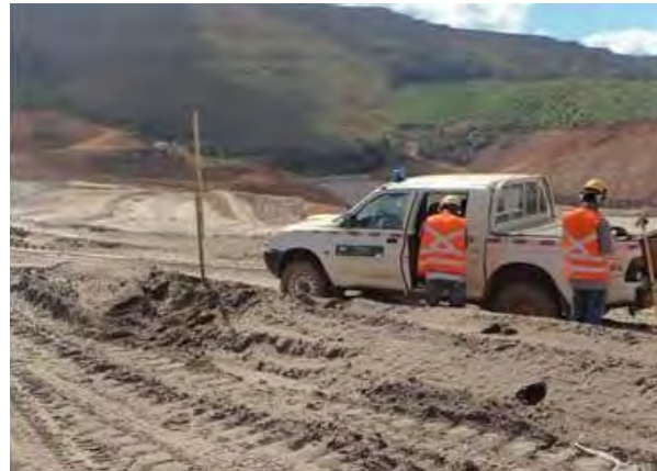
13-D: Photo from weekly report, week of August 9, 2015: "Topographic milestones between piles 10 and 20, to the 897.00 m elevation."
