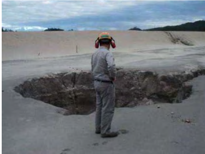
Figure K2-10 Sinkhole over Secondary Gallery, November 25, 2012 from April, 2013 ITRB report
