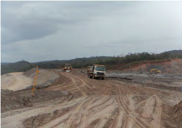
16-A: Photo from weekly report, week of September 6, 2015: "Heightening of Dike 1's crest to the 898 m elevation."
