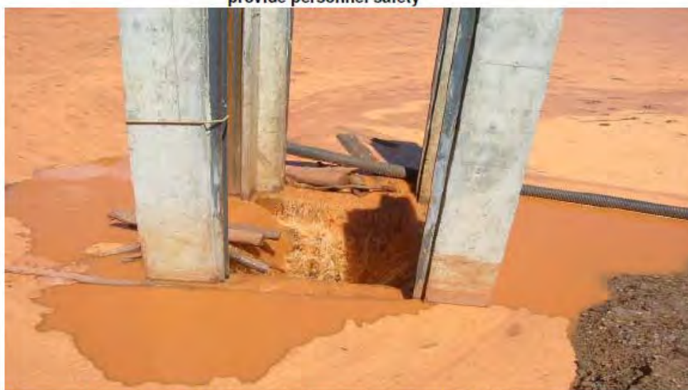
Photo 4 - Intake (from prior inspection) showing debris entry
