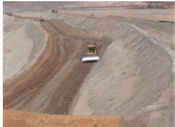
20-C, D: Photo from weekly report, week of October 11, 2015: "Heightening of the berm downstream from the left-side abutment, to ensure a safe height (5.00 m) between banks 895/900 m, allowing the heightening to proceed."
