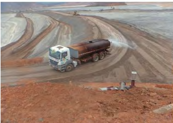
16-C, D: Photo from weekly report, week of September 6, 2015: "Tanker truck and power grader to water and level the 898.00 m crest, near the left-side abutment channel."
