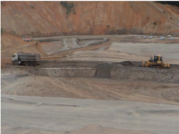
20-B: Photo from weekly report, week of October 4, 2015: "Construction of a dike for tailings to be discharged hydraulically at the return of the original axis, left-side abutment of Dike 1."
