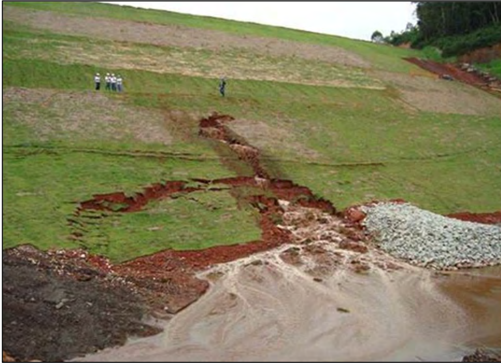
Figure 2-6 Internal erosion effects on downstream slope of Dike 1
