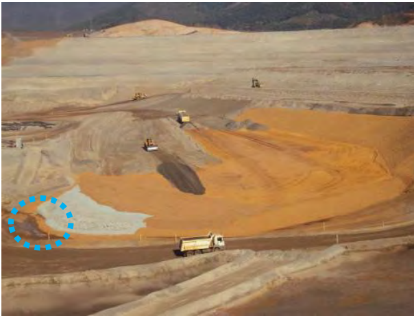
14-E: Photo from VOGBR report dated July 21, 2015 to August 20, 2015 [21] showing left setback. Dashed blue line around ponded water.
