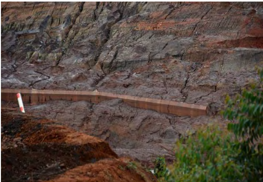
Figure K2-11 Post failure remnant of Secondary Gallery (March 1, 2016 photo)
