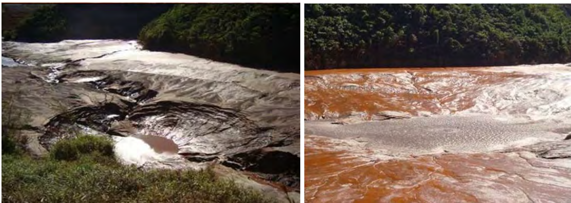
Figure K2-12 Tailings depression resulting from break in Main Gallery [25]
