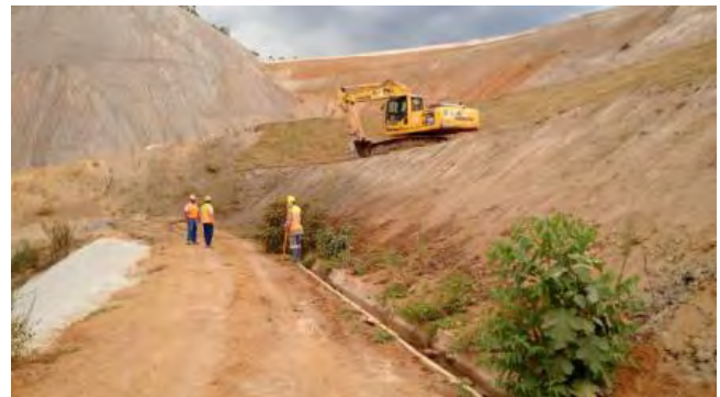
January, 2015 construction photo showing the beginning of stripping for placement of drain material on the slope [35] .
