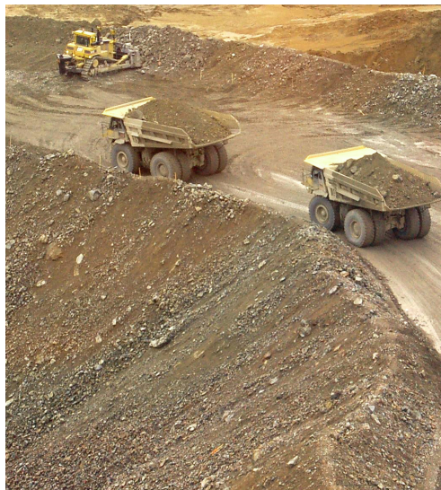
Haul trucks lined up to build a rock berm to hold back tailings in the TSF so that the breach could be repaired safely
