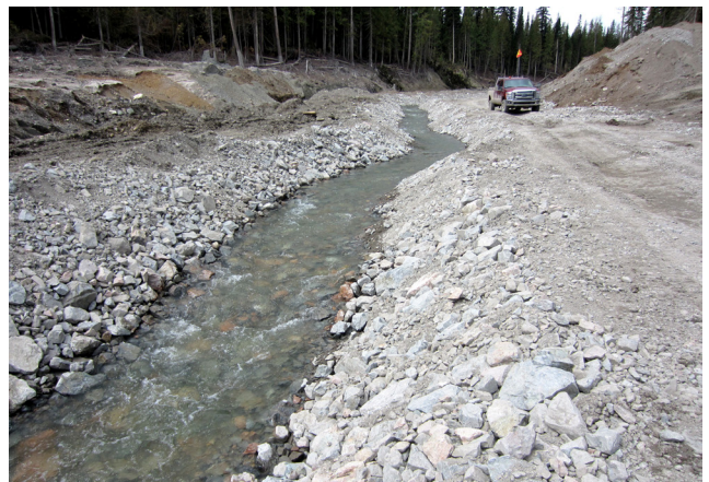
Photo 2: Mean Annual Flow channel construction
