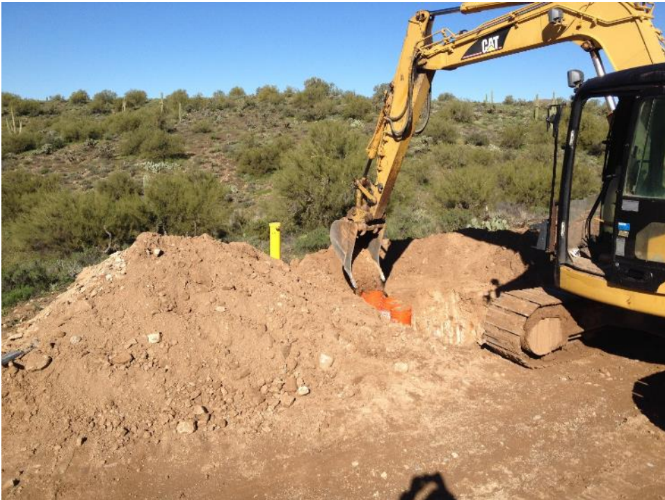
Photo II-22 TP17-35 - Pile of excavated material and buckets being filled with sample. (Mar. 1, 2017)
