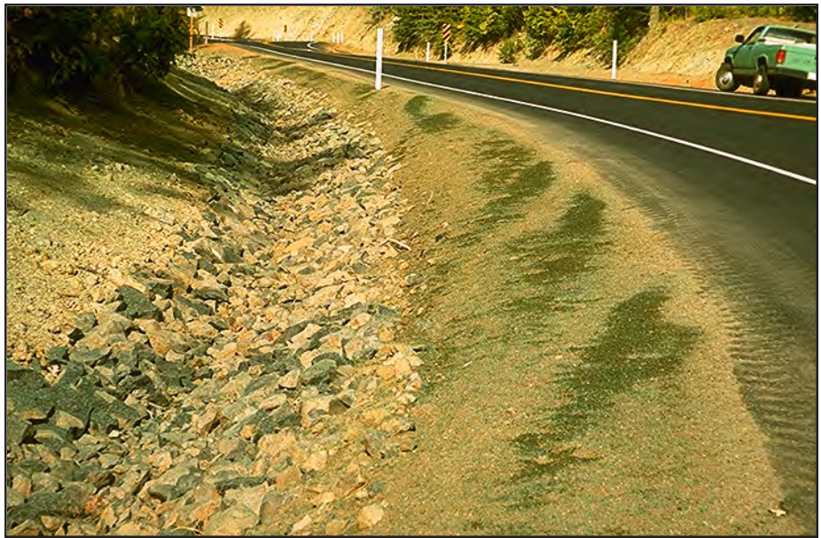
Photo 3.5 Maintain roads and drainage features to withstand major storm events with minimum erosion, such as with armored ditches that are kept clean.
