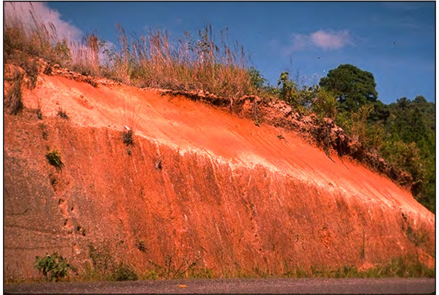
Photo 11.2 Construct cut slopes at a 3/4:1 or flatter slope in most soils for long-term stability. In well-cemented soils and rock, a 1/4:1 cut slope will usually be stable.
