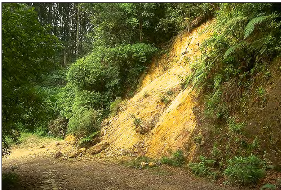
Photo 11.1 Over-steep slopes, wet areas, or existing slide areas can cause instability problems for a road and increase repair and maintenance costs, as well as sediment production.
