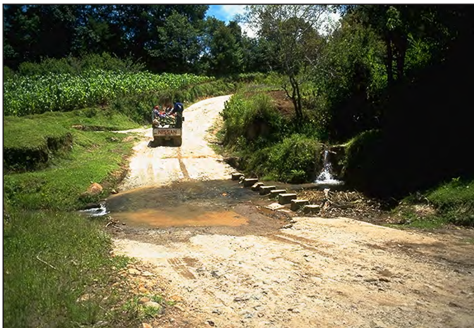
Photo 9.1 Use armored low-water crossings, fords, or drifts as often as possible to cross low flows in broad, shallow natural drainages, thus avoiding the use of pipes. Note that part of this reinforced driving surface needs repair.
