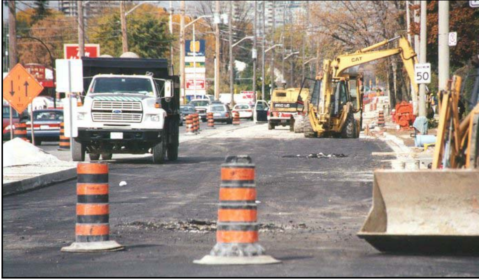
Figure 7.5. Shifting of traffic to accommodate construction. (Photo #1261)
