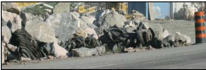
Figure 7.21 Blasting mats constructed with black tires (in foreground of photo) (Photo #261)
