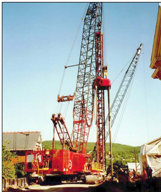
Figure 5.24 Pile driving operation (Photo #856)
