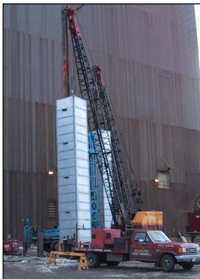
Figure 7.16 Examples of pile driver shielding and dampening (Photos #1277, #1281 & #1308)
