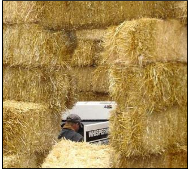
Figure 7.20 Straw bail enclosure for stationary equipment (Photo #58)
