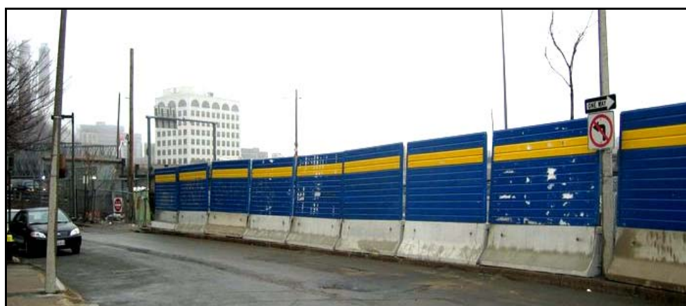
Figure 7.31 Temporary barrier of plastic material (Photo #194)
