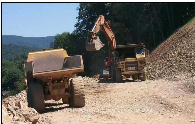
Figure 5.25 Rock excavation operation (Photo #981)
