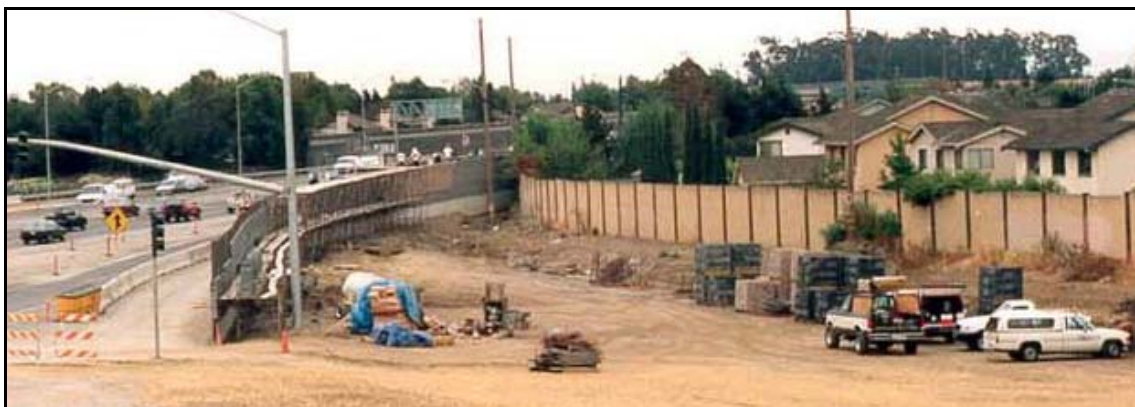
Figure 7.28 Existing noise barrier left in place until replacement noise barrier is constructed (Photo #483)
