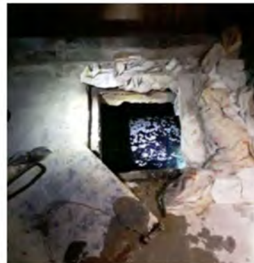
Photo 2. Government Springs, uncovered spring box in the back of the bunker. The box is plumbed into the nearby ranch house. September 2019
