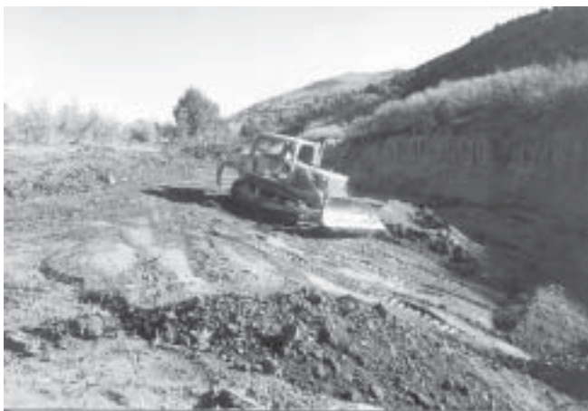
Figure 36 —Three-way dozer reshaping a streambank.
