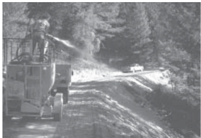
Figure 33 —Hydroseeding roadcuts and fills.
