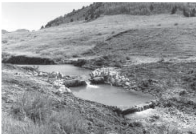
Figure 8 —Channel reshaping and construction of impoundments may be required to stabilize stream channels prior to seeding and planting.
