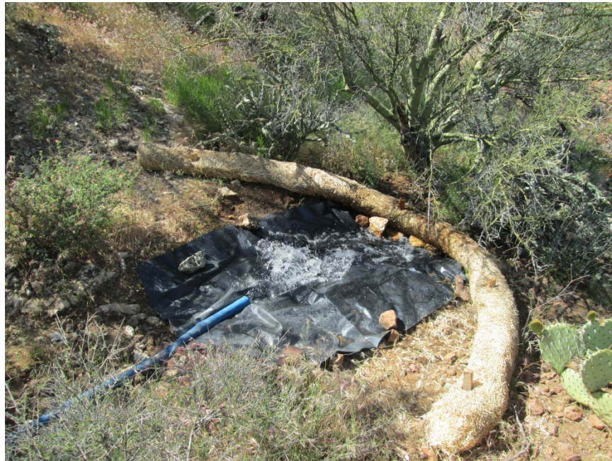
Plastic sheeting and straw wattles used as erosion controls at DS16-07
