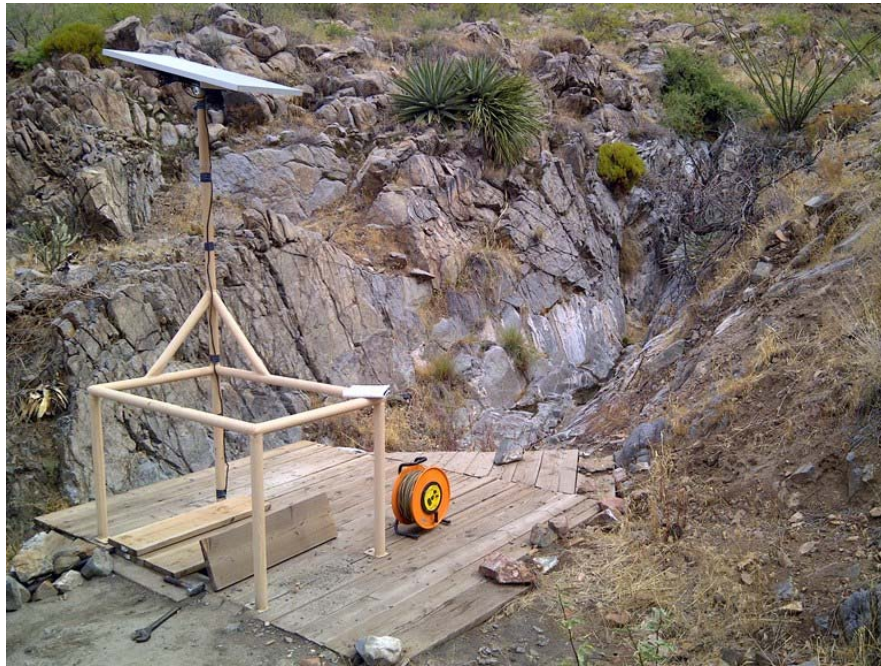
Photograph A-1. Spring sump with solar panel powered pump
