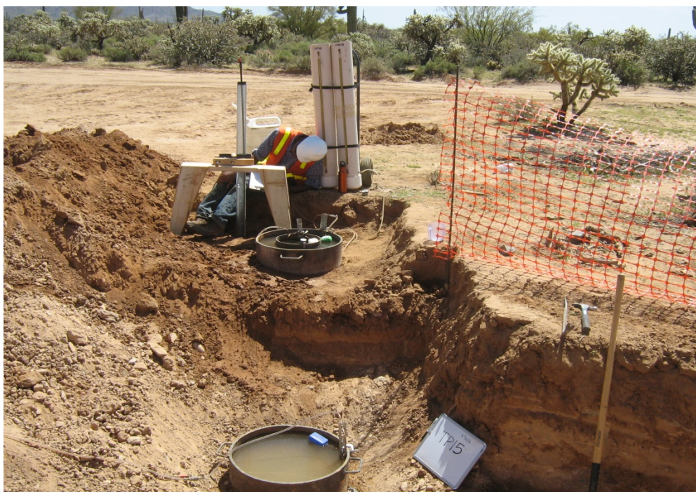
Double-ring infiltrometer, single-ring infiltrometer, and constant-head permeameter tests conducted in Test Pit 15.
