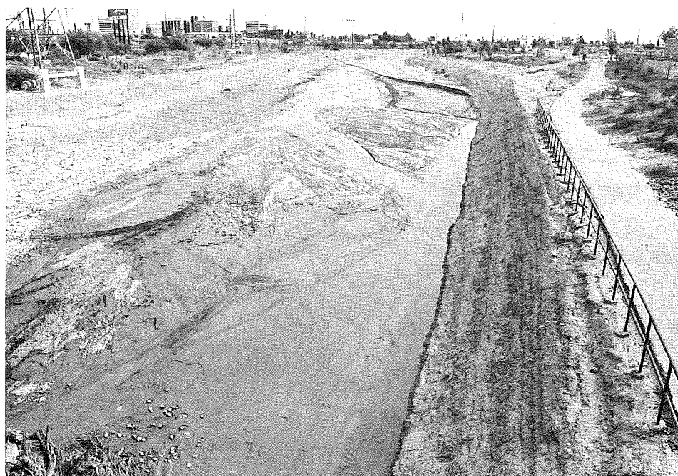
Figure 6a. Same area as Figure 1 after passage of major flow. Right bank with railing is undamaged soil cement. Photo by Peter Kresan.
