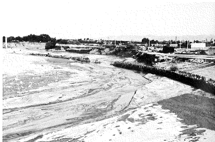
Figure 7b. Rock-and-wire-mesh bank-protection device breached and overtopped in October 1983. Looking north along Santa Cruz River from bridge at W. Grant Road. Photo by H. Wesley Peirce.
