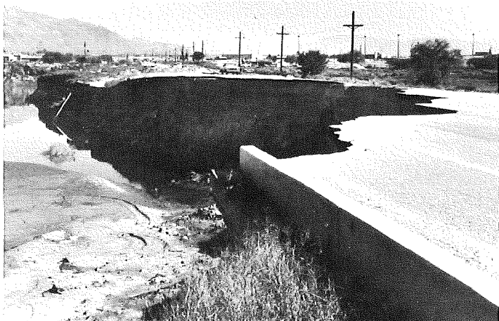
Figure 3a. Ina Road undercut by water from adjacent Santa Cruz River. Looking northeast. Photo by Ken Matesich.
