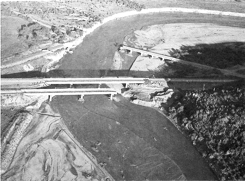
Figure 2a. Severe bank-cutting along the Santa Cruz River near I-19 and San Xavier Road. Looking northwest. Bridge segment nearest viewer collapsed when support washed out. Bridge in distance did not fail. Bank retreated from west end of bridge to present position. Distance between bank and midstream end of bridge is measure of amount of bank erosion that occurred. Photo taken on October 9, 1983 by Peter Kresan.
