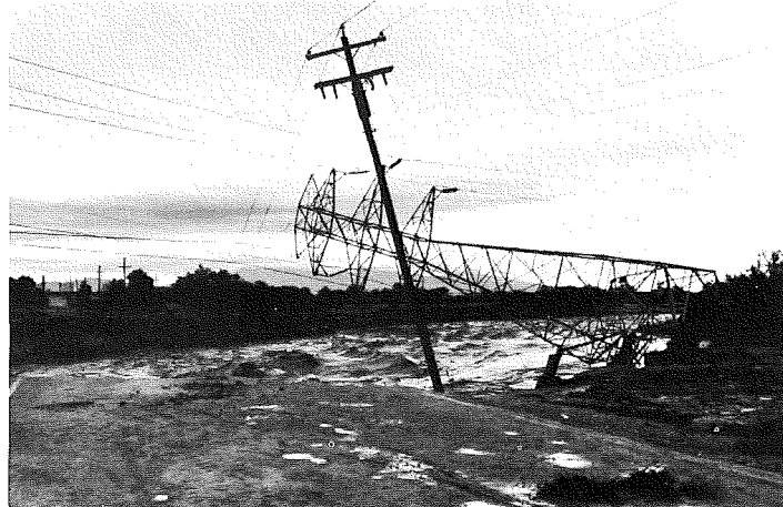
Figure 3b. Wipeout of bridge and utility tower at Sunset Road crossing of Santa Cruz River. Looking southeast. Photo taken on October 2, 1983 by Steve Reynolds.
