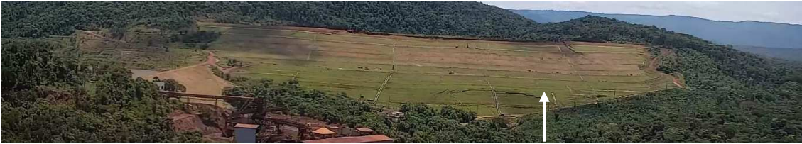
Figure 6: Bulging Above the Toe of the Dam Approximately One-Third in from the Left Abutment (Right Side of Photograph), Initiated About 0.2 s After the First Observed Deformation at Crest
