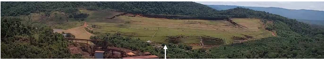
Figure 7: Continued Settlement of the Crest and Bulging Above the Toe with Water Erupting Above the Toe Toward the Right Abutment (Left Side of Photograph) About 5.5 s After the First Observed Deformation at Crest
