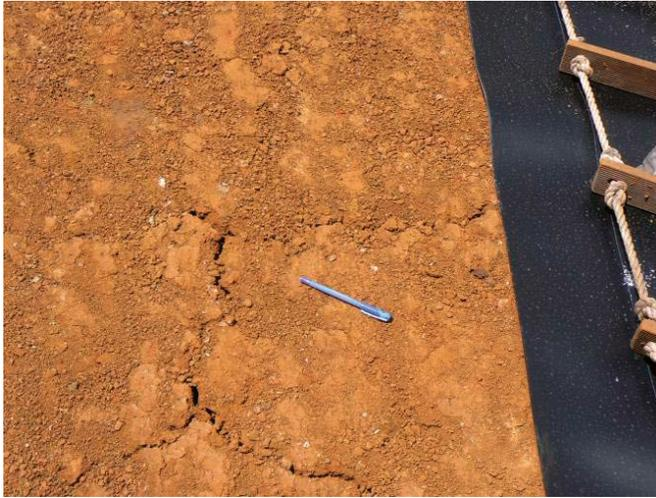
**Fig. 3.** Compacted clay liner (forming part of a composite liner) that has desiccated (photo courtesy of P. Davies).
