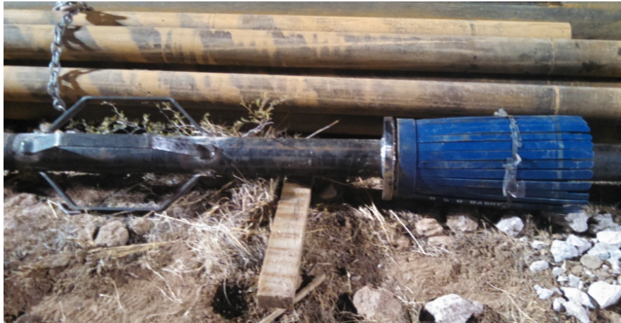
Cement Basket and Centralizer on 4-1/2-inch OD steel casing installed at HRES-21
