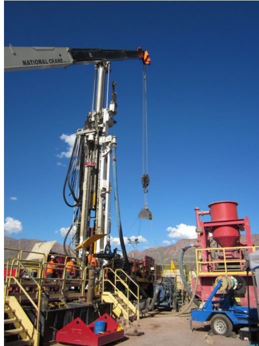
Grouted piezometer installation at DHRES-16
