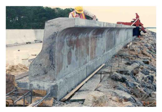
Figure F-1. Example 1: curved parapet wall, maximum protection against wave action
