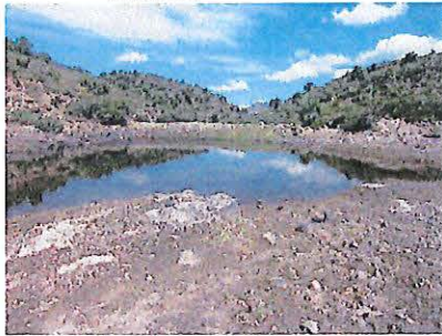
Figure 1: Walt Tank in satisfactory condition NAD12S E498507 N3686357
