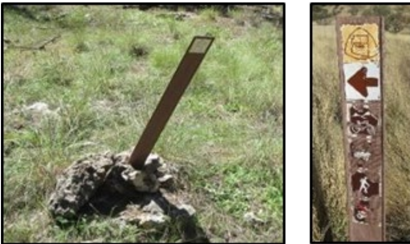
Figure 26. Examples of fiberglass signage improperly installed or in poor condition
