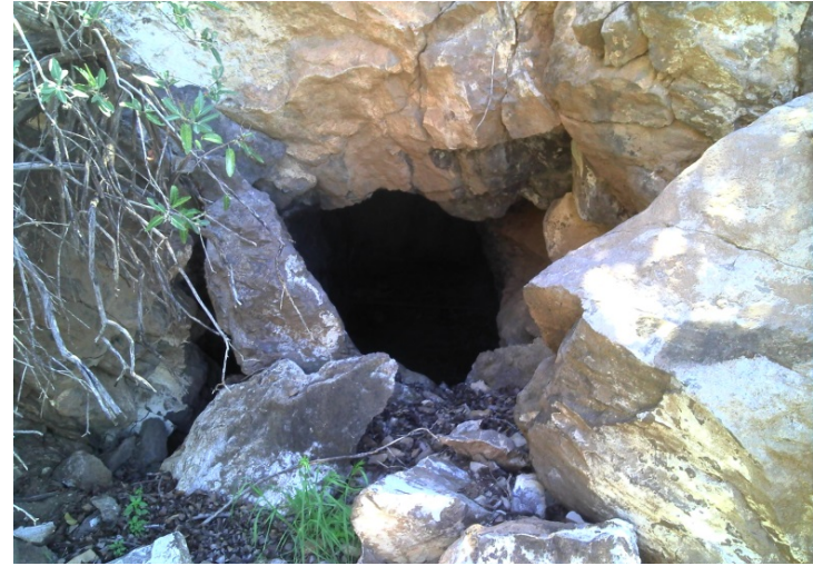
Photo 10. Mine adit measuring 17' long x 7' wide x 8' tall; opening measuring 6' x 3'.
