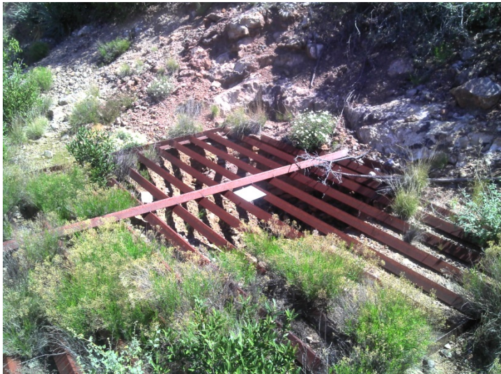
Photo 3. Iron gate on partially filled-in shaft, shaft appears to be 6' x 6' x 3'.
