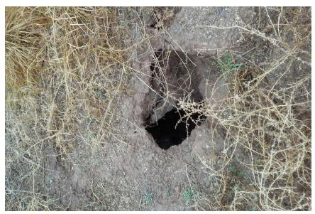
**Photo 46.** Holes in ground, suspected to have resulted from subsidence; no evidence of buried debris visible.
