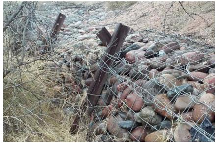
Photo 12. Rock gabion berm.
