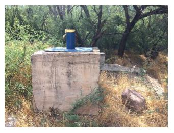
Photo 22. Well structure with locking cap on casing.
