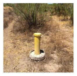
Photo 13. Well casing with locking cap.
