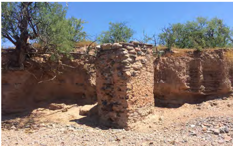
Photo 3. Rock-lined well; view from within the channel.
