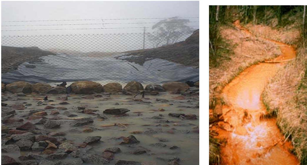
Figure 52: Dam failure and leakage
