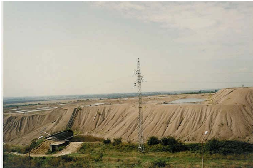
Figure 7: Erosions cracks on the side of heap leaching piles
