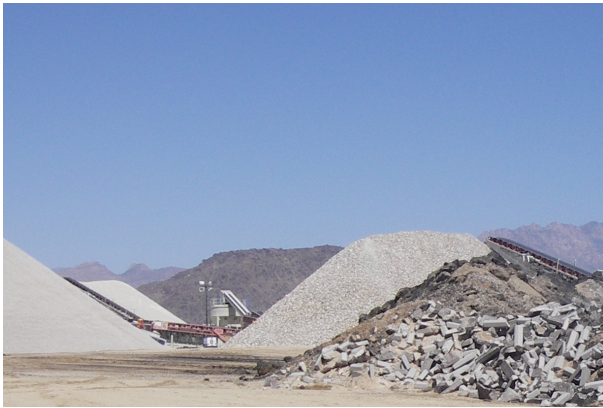
Figure 9.4 Batch plant and crusher.
