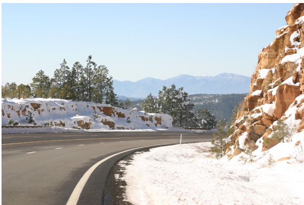
Figure 11.9 Snow removal should ensure inert materials do not interfere with drainage structures as the snow melts.
