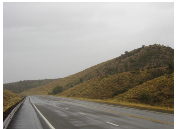
Figure 4.17 Rounded minibenched cut slopes blend into the native landscape.
