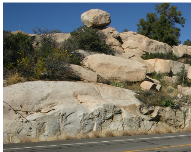
Figure 4.23 Visible scars from drill-hole traces.
