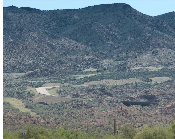
Figure 4.28 Obliteration of old highway corridor at the left and above new highway alignment.
