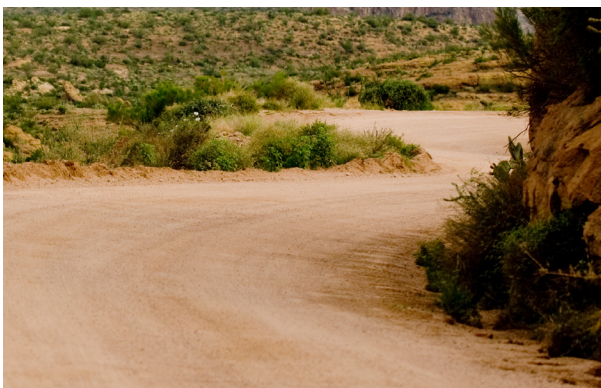
Figure 11.7 Maintenance of unpaved roads include installation of BMPs.
