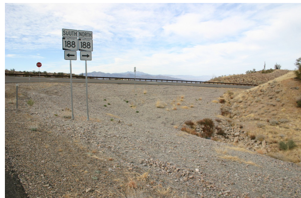
Figure 6.8 Area where runoff will intercept a cut slope.
