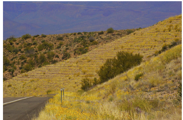
Figure 7.4 Mini benching allows for more water retention thus giving seeds a better chance to take hold.
