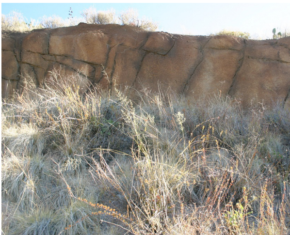
Figure 4.29 Retaining wall colored to integrate into surrounding landscape.
