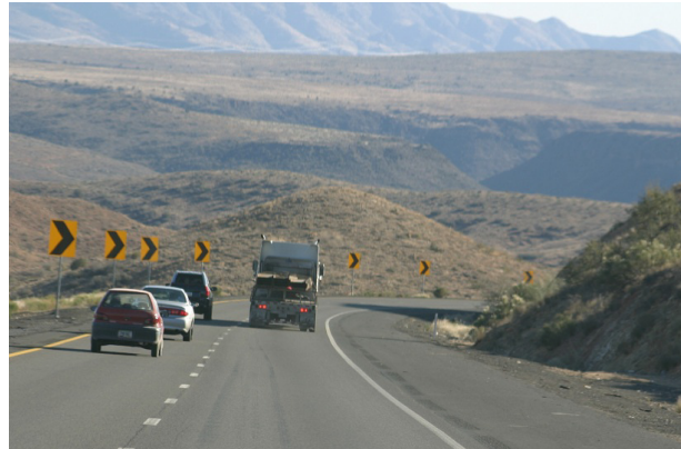
Figure 3.3 Reducing speed by designing with steeper grades.
