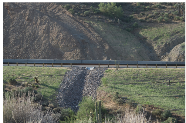
Figure 6.9 Embankment curb opening into a spillway.
