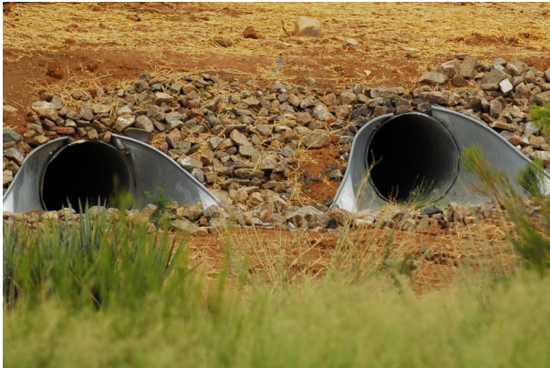
Figure 6.10 Flared end-section of a culvert.
