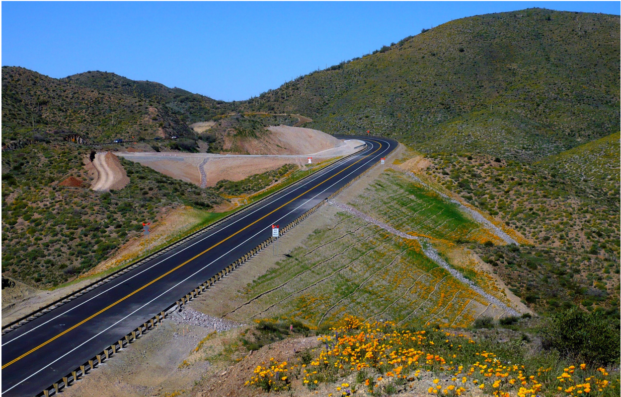
Figure 10.2 Seeding is a way in which soils can be stabilized after construction activities.
