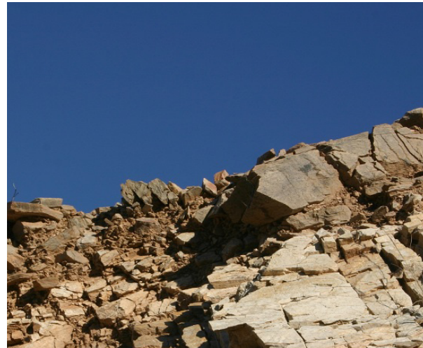
Figure 4.22 Highly fractured, unorganized cut.
