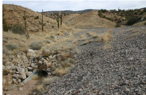
Figure 6.7 Erosion protection at cut-to-fill transition.
