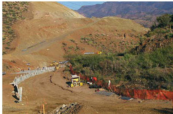
Figure 10.4 Barrier marking materials may be required for areas to be left undisturbed.
