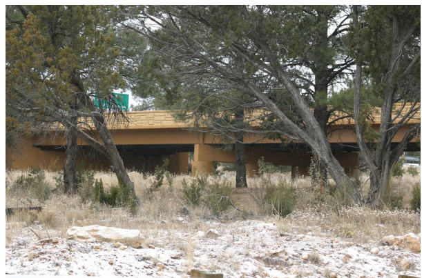
Figure 3.8 Cover beneath bridges is important for animal movement.
