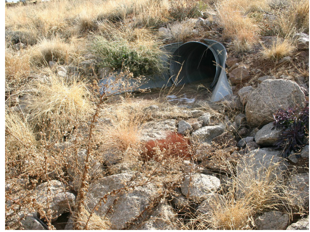
Figure 3.12 Small pipe culvert.
