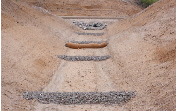
Figure 6.4 Rock check dams reduce runoff velocity.
