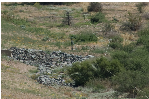
Figure 10.3 Staking of clearing limits is required prior to clearing.
