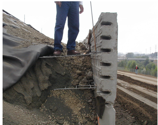
Figure 4.30 Mechanically Stabilized Earth (MSE) wall.
