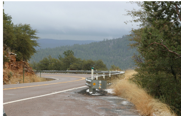
Figure 1.7 Highway through the forest.
