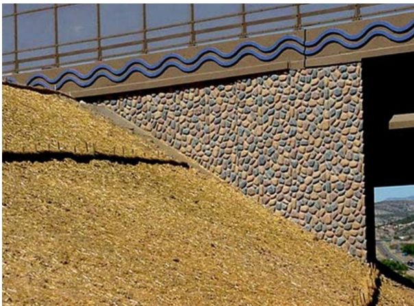
Figure 4.35 Reinforced concrete, typically cast-in place can utilize form liners.
