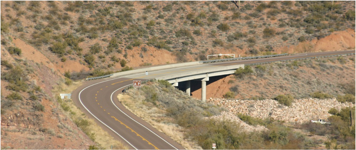
Figure 5.2 Bank protection of rip rap to control damage to bridge structure and embankment.
