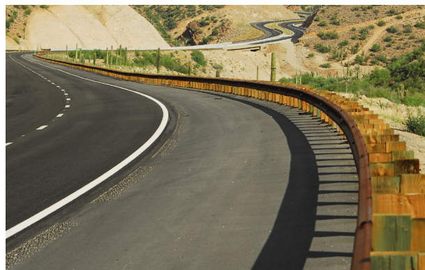
Figure 11.8 Non-specular steel roadside barrier.
