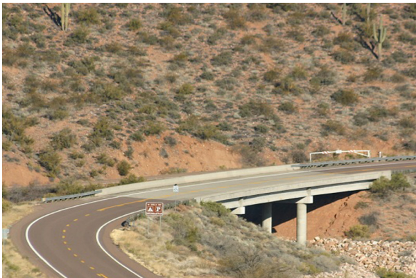
Figure 5.9 Concrete I-Beam construction.
