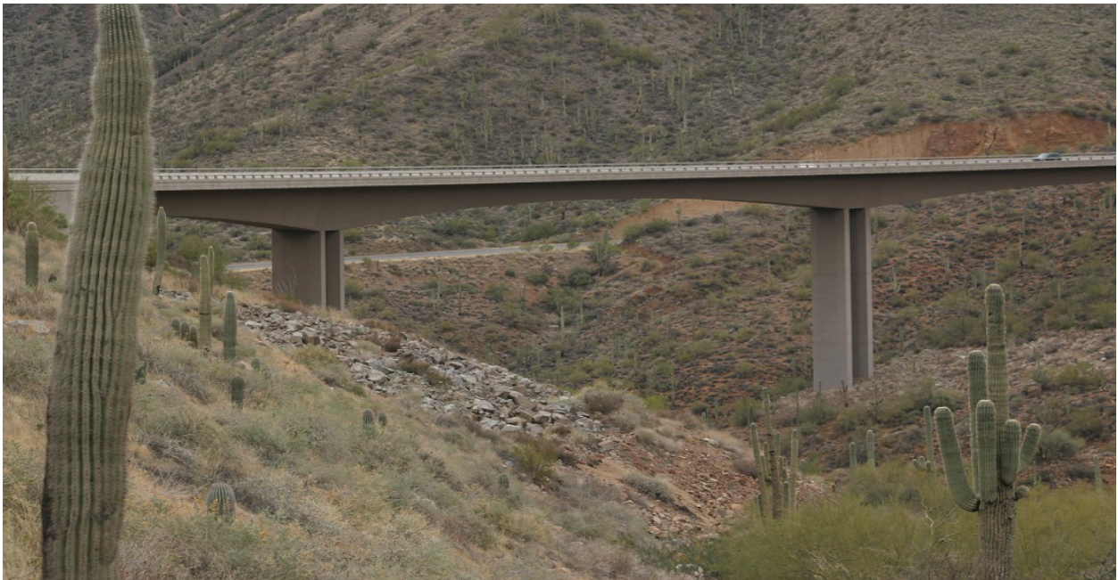
Figure 5.12 Cast-in-place segmental box bridge design.
