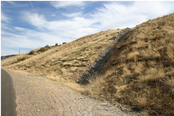
Figure 6.6 Slope ditch installed to intercept sheet flow and convey concentrated flows.
