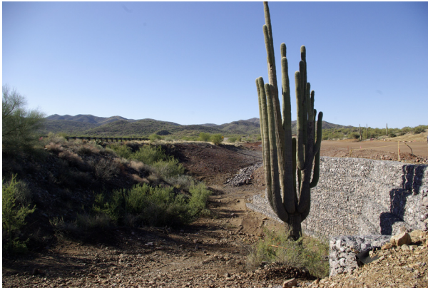
Figure 7.2 Beautiful, large saguaro protected by gabion wall..
