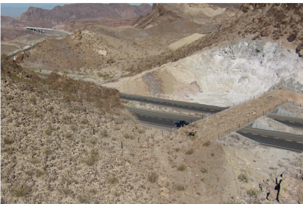
Figure 3.6 Planned wildlife overpasses for Big Horn Sheep on US 93, construction 2008 - 2009.
