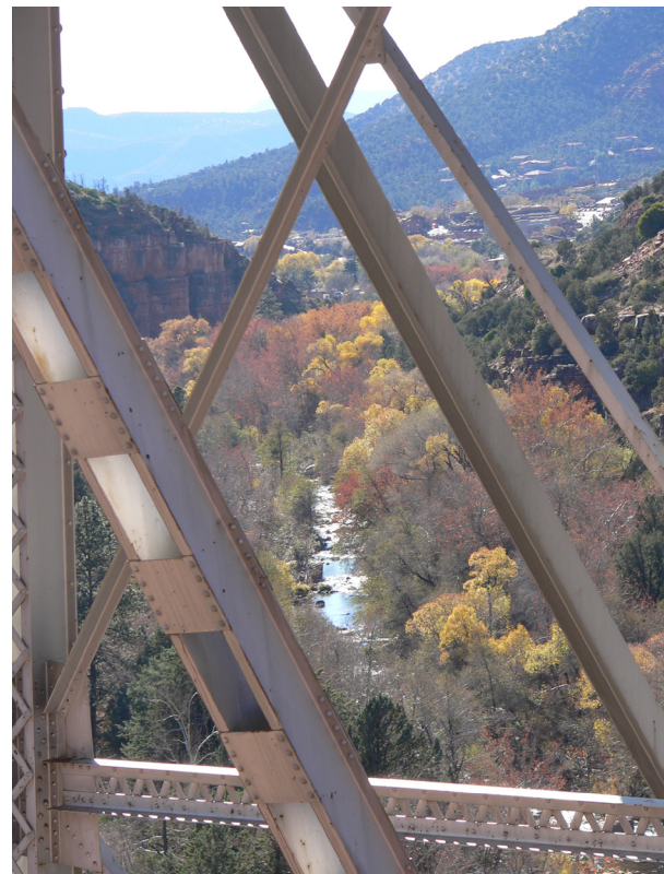
Figure 2.5 Steel bridge over riparian habitat.
