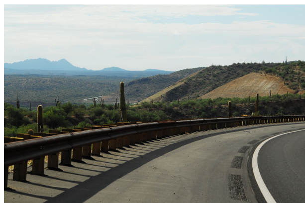
Figure 4.6 Roadside barrier of steel with wood posts.
