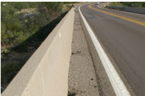
Figure 5.5 F-Barrier (Jersey barrier).
