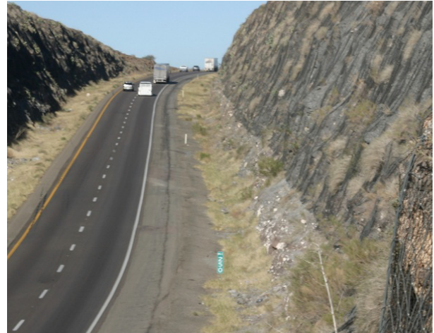
Figure 4.26 Mesh draped over slopes for rockfall containment.
