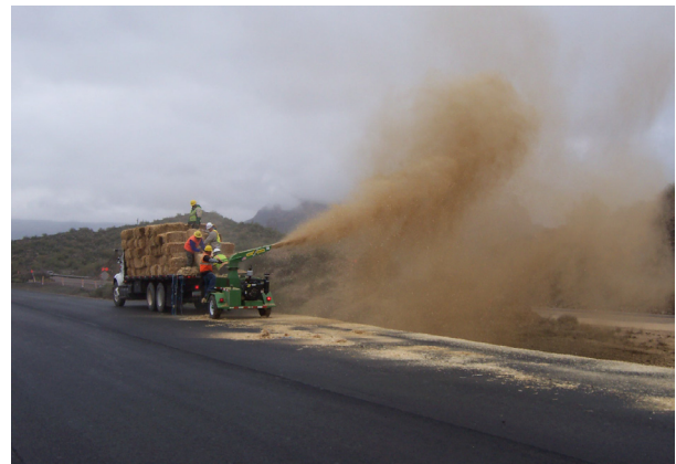
Figure 7.8 Straw provides superior erosion control and insulation against heat and moisture loss.
