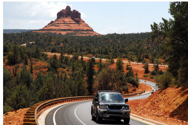
Figure 2.8 Views of the roadway.
