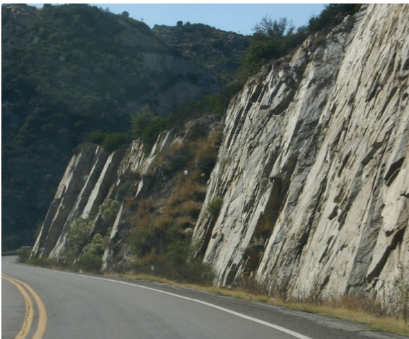
Figure 4.21 Cuts should create irregular ledges and sheer faces.
