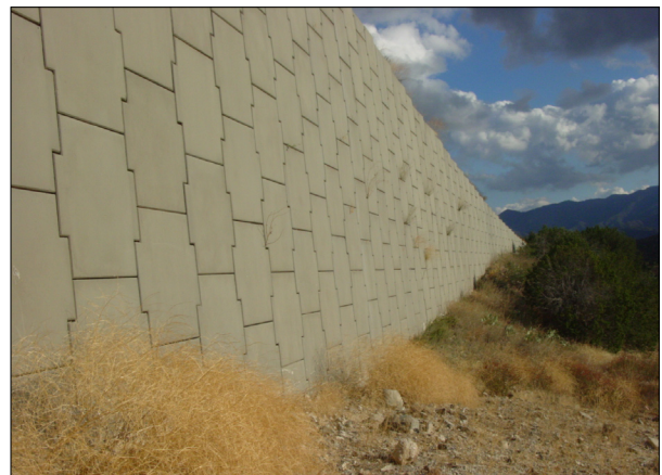
Figure 4.31 MSE wall face.
