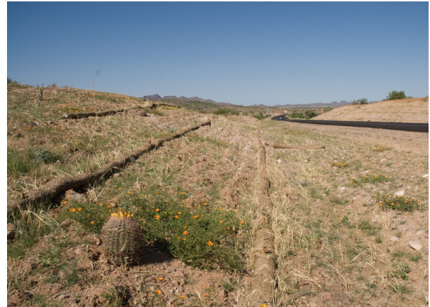
Figure 4.16 Rippling improves moisture infiltration and revegetation success.
