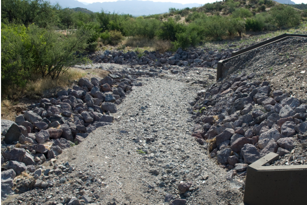
Figure 6.11 Riprap helps to reduce erosion at outfalls.
