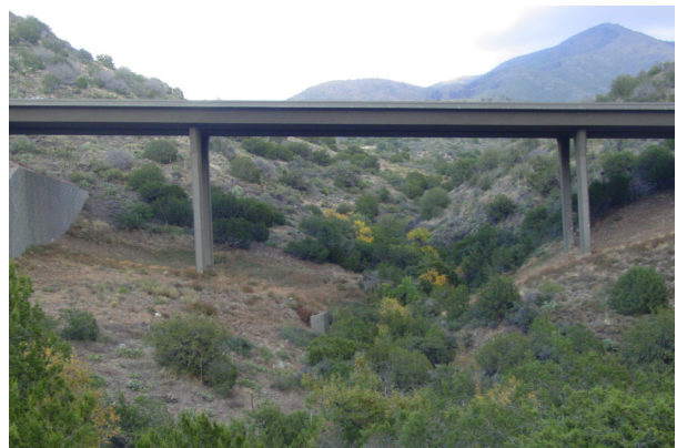
Figure 5.11 Cast-in-place post-tension box girder design.
