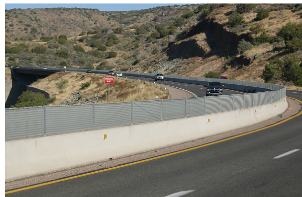
Figure 5.6 F-Barrier with semi-transparent headlight screening.
