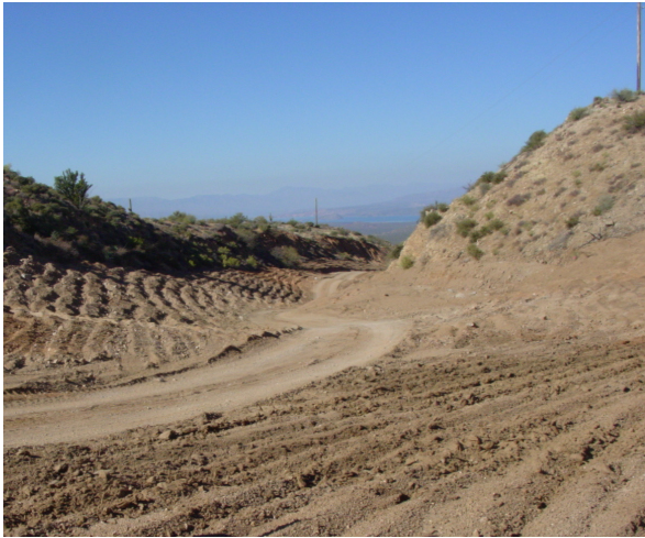
Figure 4.13 Example of ripping.
