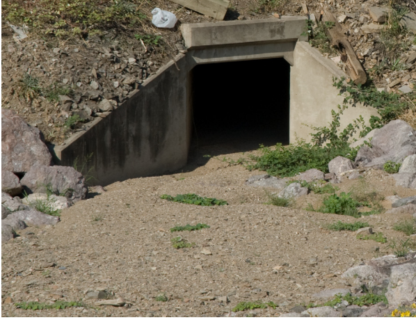
Figure 3.11 Culverts should be free of obstacles.
