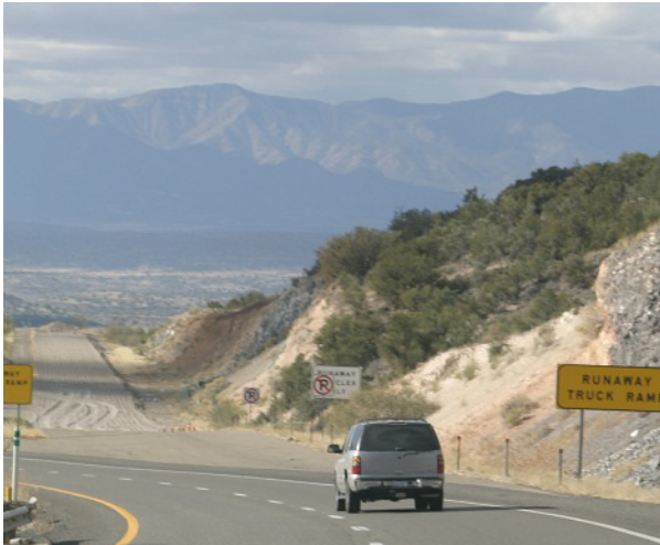
Figure 4.7 Truck escape ramp.
