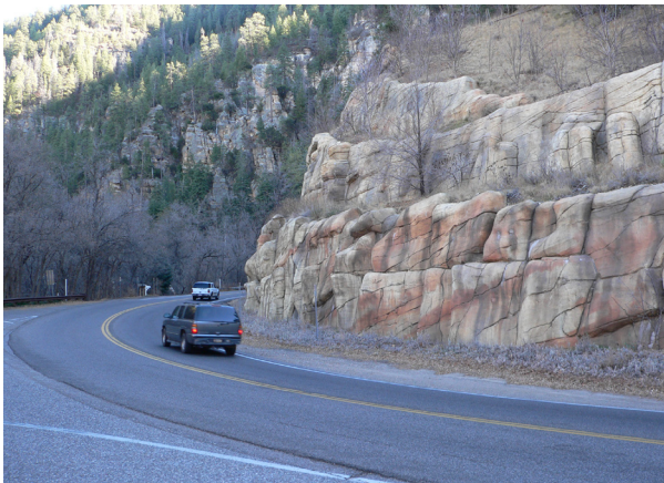
Figure 4.34 Soil nails to mimic natural rock outcroppings.
