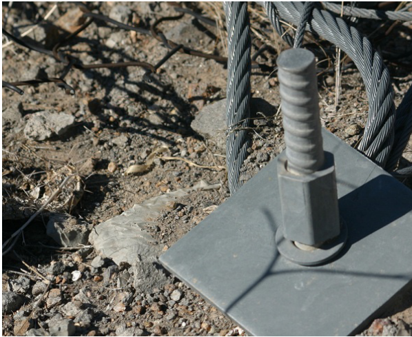
Figure 4.24 Mesh attached to rebar.
