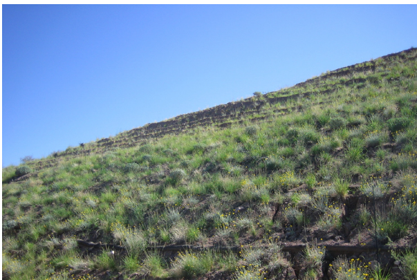
Figure 7.6 Successful revegetation using seeding on a cut slope.
