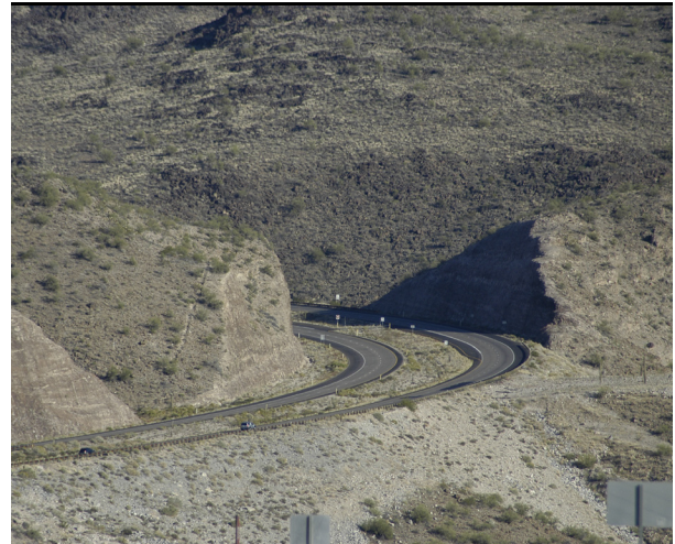
Figure 4.8 Fill slope made using waste material.
