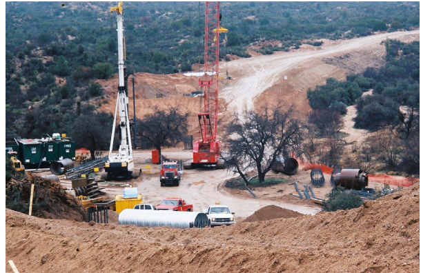
Figure 5.10 Pads for cranes.
