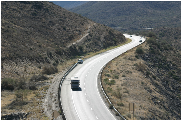
Figure 3.2 Highway laying lightly upon the natural terrain.
