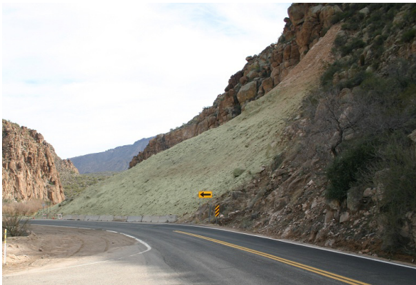
Figure 7.7 Slope on the right has been hydroseeded.
