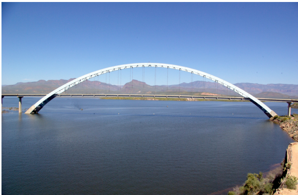
Figure 5.8 Steel arch bridge with concrete deck.
