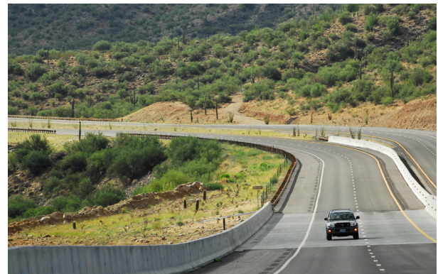
Figure 4.2 New highways have wider cross-sections and flatter profiles.
