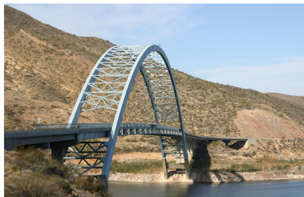
Figure 5.4 Longer bridges have less impact to waterways.
