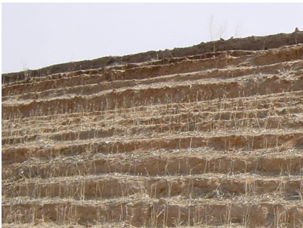
Figure 4.15 Mini benches increase water retention.
