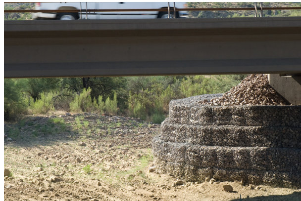
Figure 6.2 Gabion baskets used for bank protection.
