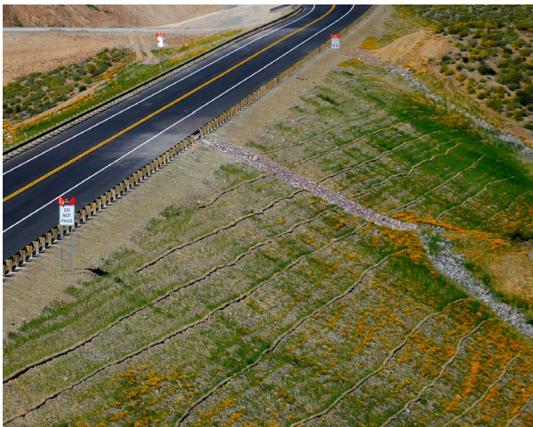
Figure 4.14 Seed, mulch and wattles applied on steep slopes.
