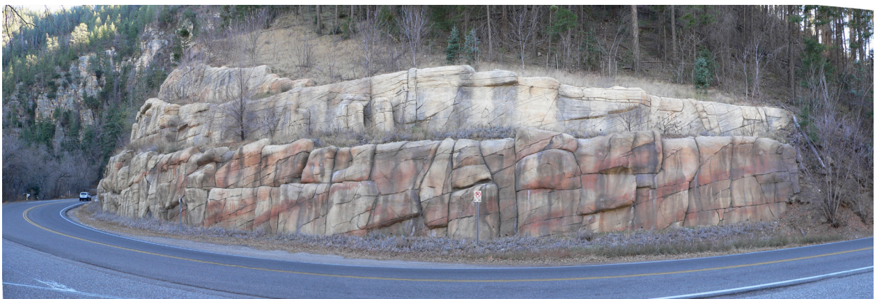
Figure 4.25 Shotcrete facing formed and colored to mimic rock outcropping.
