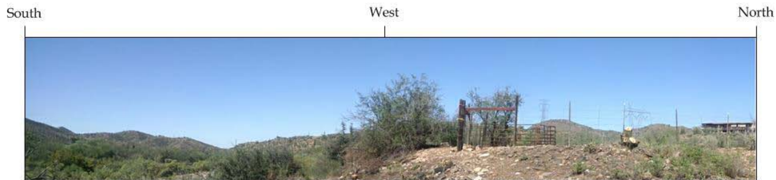
Figure 19. Hewitt Station 20-Meter Tower, Facing West
