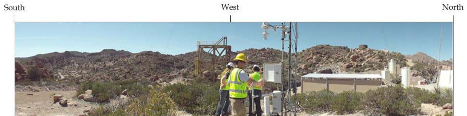
Figure 13. East Plant Station, Facing West
