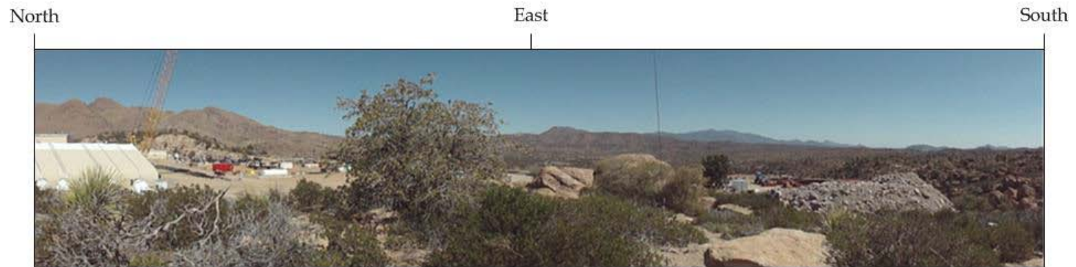
Figure 12. East Plant Station, Facing East
