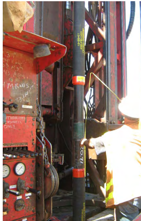
Photograph 5. Swellable packers being installed on 4-1/2-inch casing at DHRES-05B
