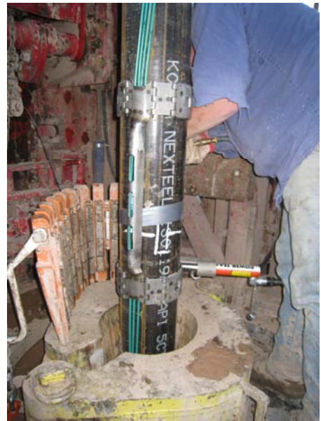
Photograph 2. Transducer protector shroud mounted on 7-5/8-inch casing
