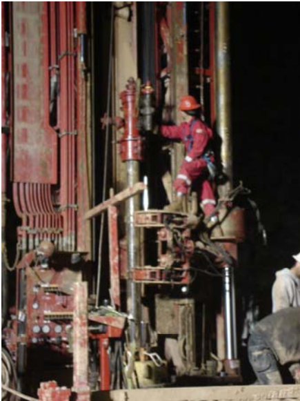
Photograph 3. Halliburton crew preparing for pressure grouting
