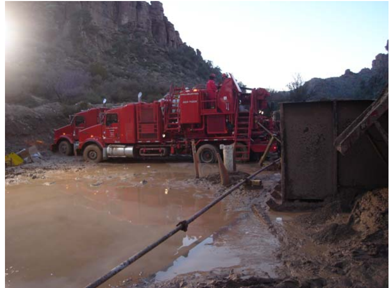
Photograph 4. Halliburton pump truck positioned for pressure grouting
