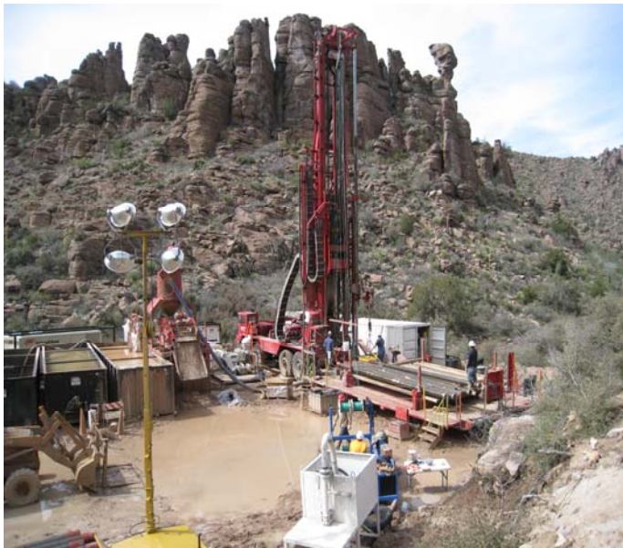
Photograph 1. Site layout during installation of 7-5/8-inch intermediate casing
