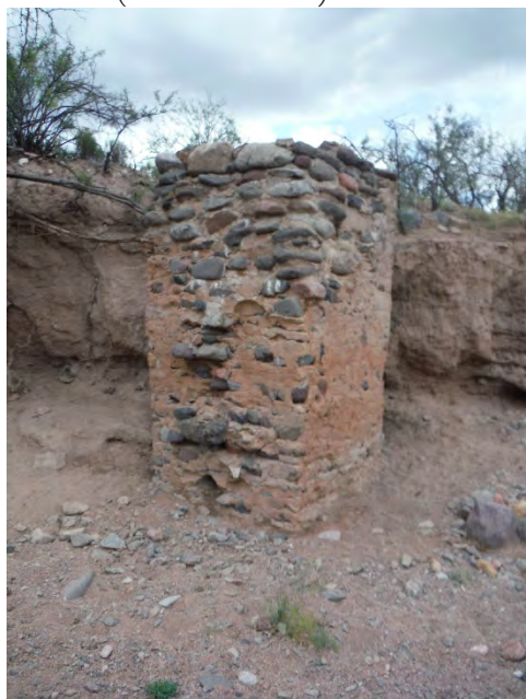
Photo 6. Rock-lined well (view from grade in wash)
