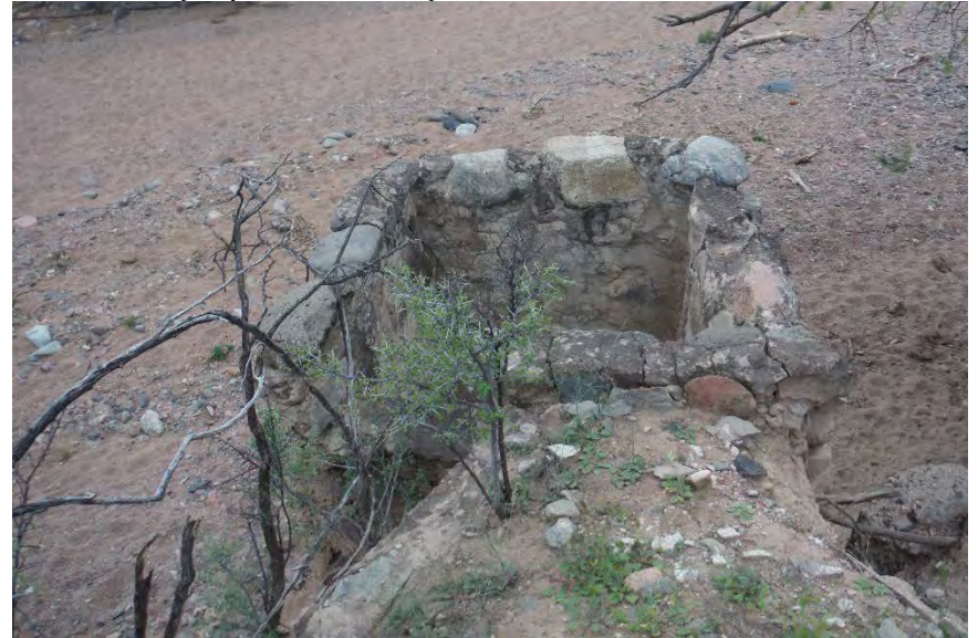
Photo 4. Rock-lined well (view from top of channel looking down)
