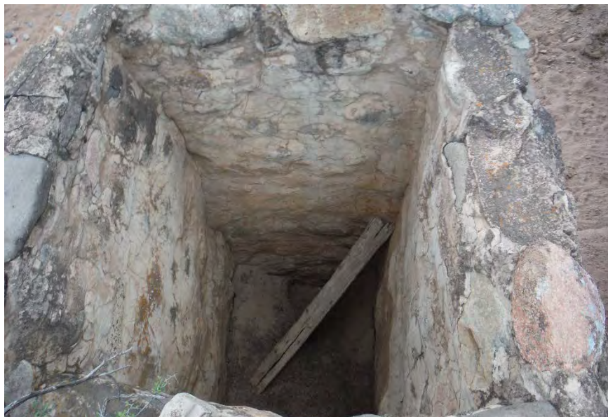
Photo 5. Rock-lined well (view inside well)
